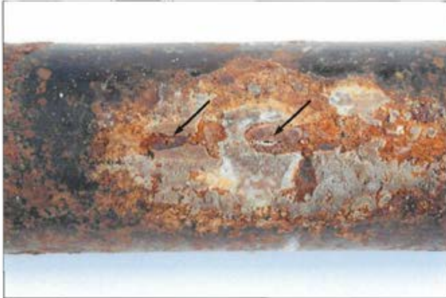
Figure 107 Main leaking defect on row 2 – tube 3 removed from bundle. Several smaller defects were found along the ERW weld.
