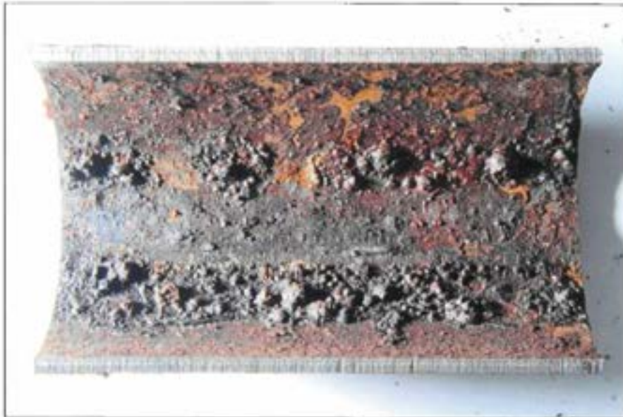
Figure 81 Corrosion found in horizontal brine pipe separated from coupling (opposite side of Figure 80 piece).
