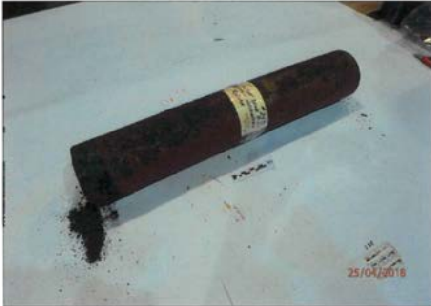
Figure 77 Horizontal brine pipe that detached from coupling.
