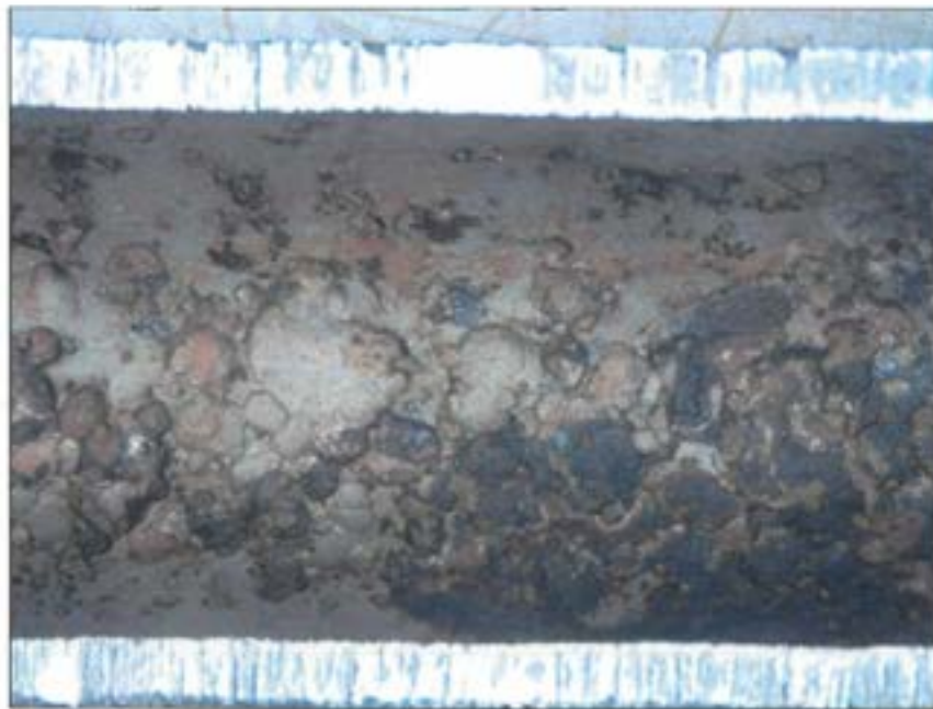
Figure 155 Corrosion damage on row 14 - tube 2 (top) after plastic bead blasting.
