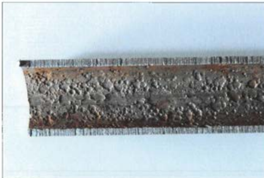
Figure 118 Typical corrosion damage found along row 2 – tube 3 approximately 12" from the leaking defect.
