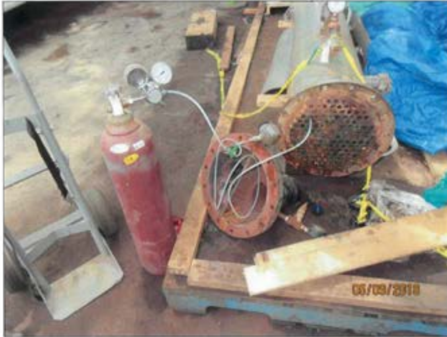
Figure 99 Pressure-test set up for steel chiller tubes.
