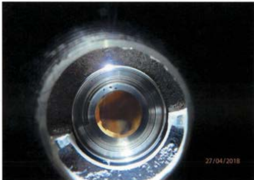
Figure 48 PRV Valve "1" internal bore. No evidence of calcium chloride is present.
