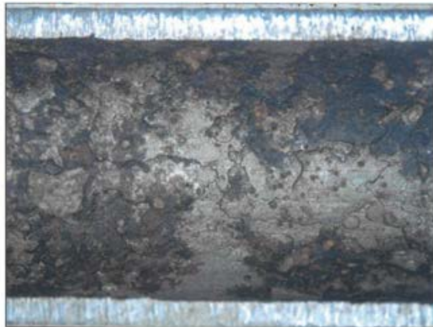
Figure 143 Corrosion damage on row 7 - tube 13 (top) after plastic bead blasting.
