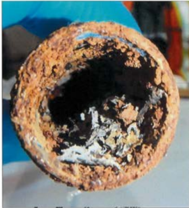
Figure 3 Partially plugged nipple on bottom end of Valve X.
