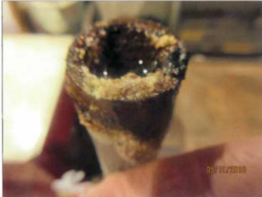
Figure 22 Water remaining at steady level in valve Z leak test.
