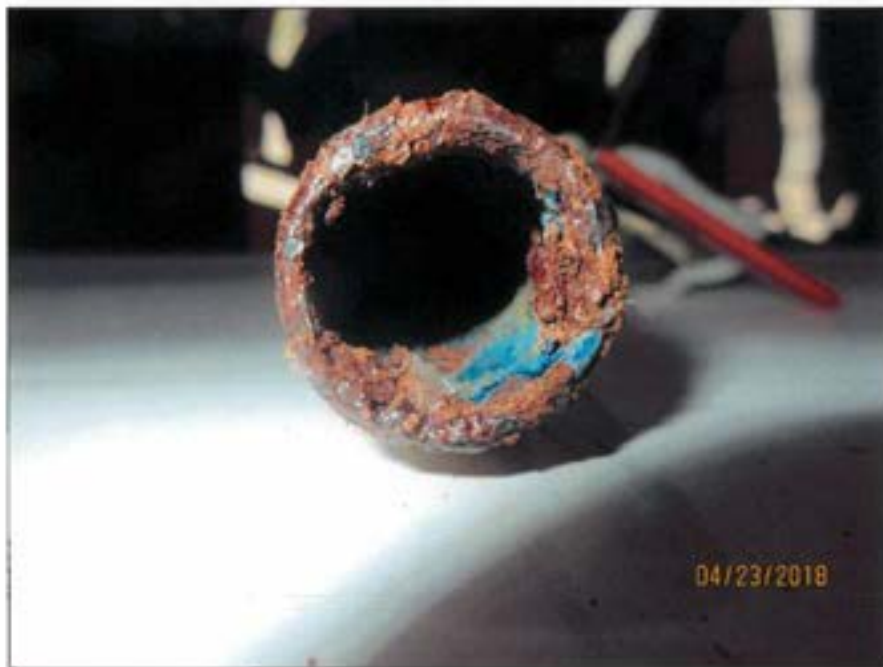
Figure 7 Corrosion products on nipple end of Valve A-3.
