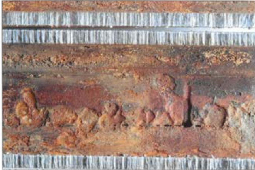
Figure 117 Closer view of leaking defect showing a line of "stitch-like" defects adjacent to the leaking defect. Nozzling effect has removed material above the leak.
