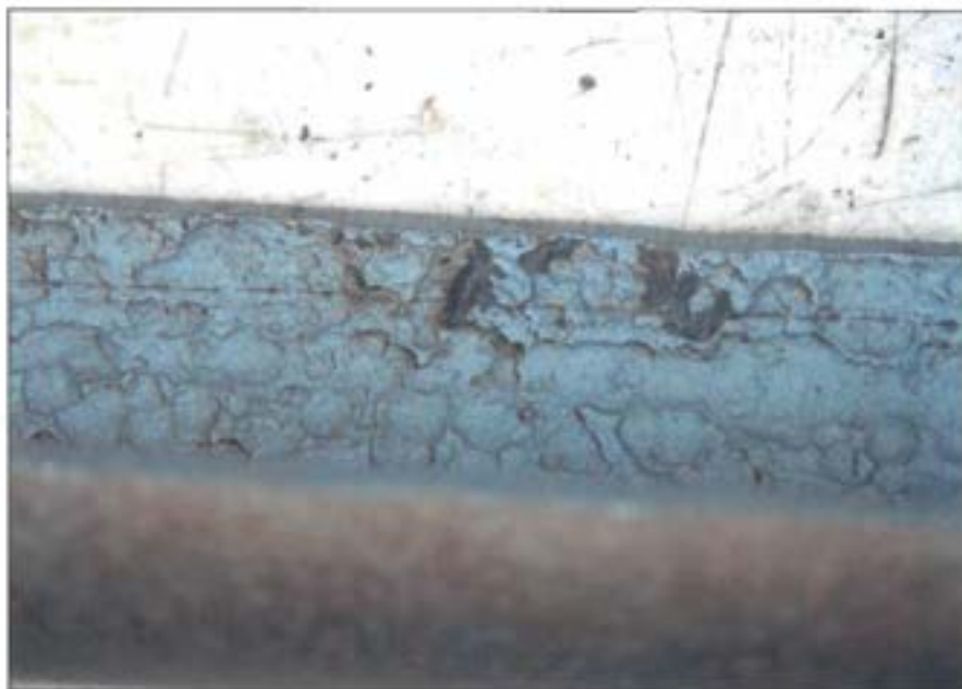
Figure 133 Corrosion damage on row 4 - tube 10 (bottom) after aluminum oxide blasting. Note "stitch-like" defect along fusion line of ERW weld.
