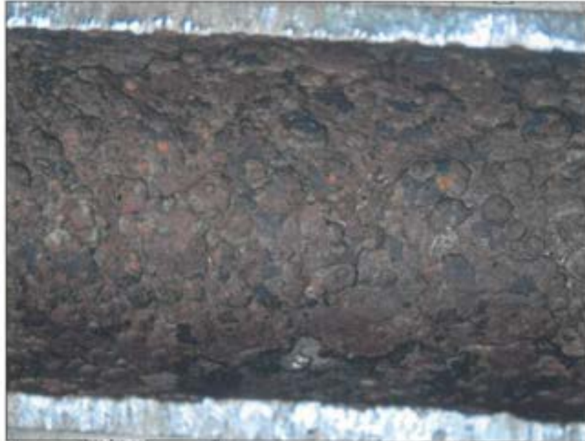
Figure 136 Corrosion damage on row 7 - tube 1 (bottom) after plastic bead blasting.
