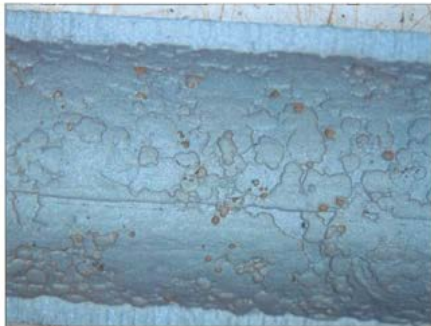
Figure 139 Corrosion damage on row 7 - tube 1 (top) after aluminum oxide blasting.
