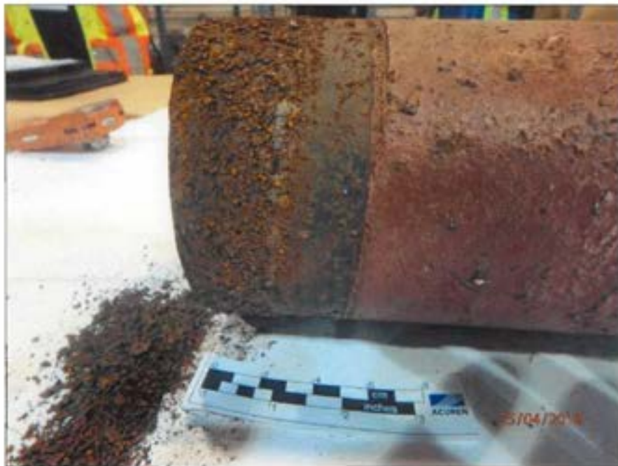
Figure 78 Corrosion found in unpainted area of separated pipe mounted within horizontal coupling.
