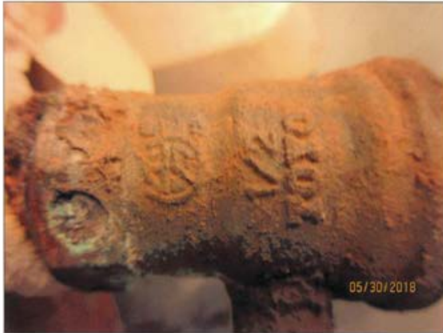
Figure 28 Markings on Valve A10.
