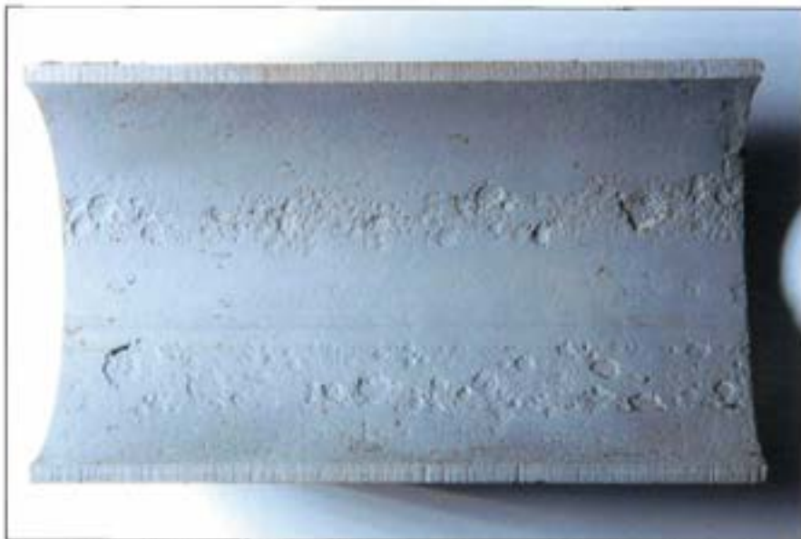
Figure 82 Sand blasted internal surface of separated horizontal brine pipe showing pitting around weld seam.
