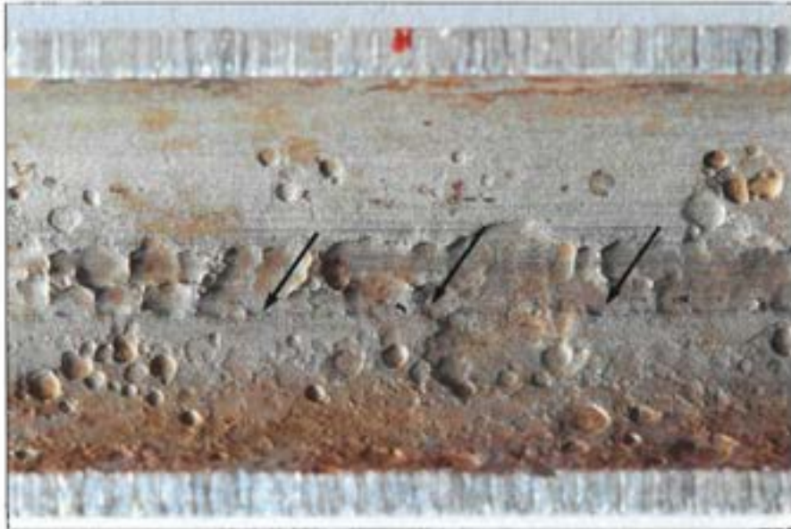
Figure 119 Closer view of corrosion damage showing a line of small, deep pits (arrows).
