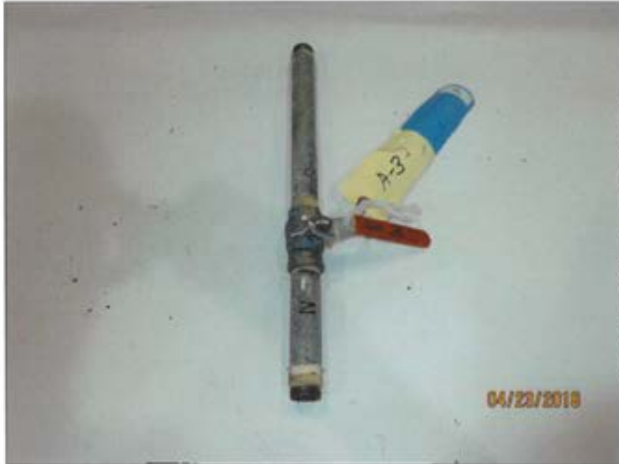
Figure 6 Overall view of Valve A-3.
