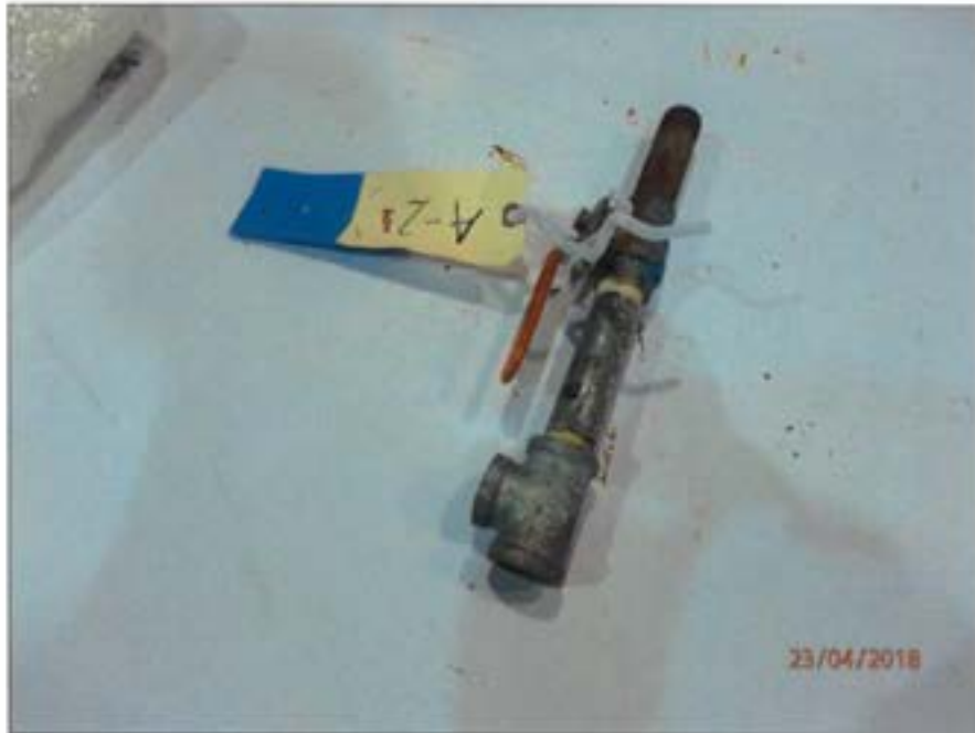
Figure 12 Overall view of Valve A-2. Handle is in open position.
