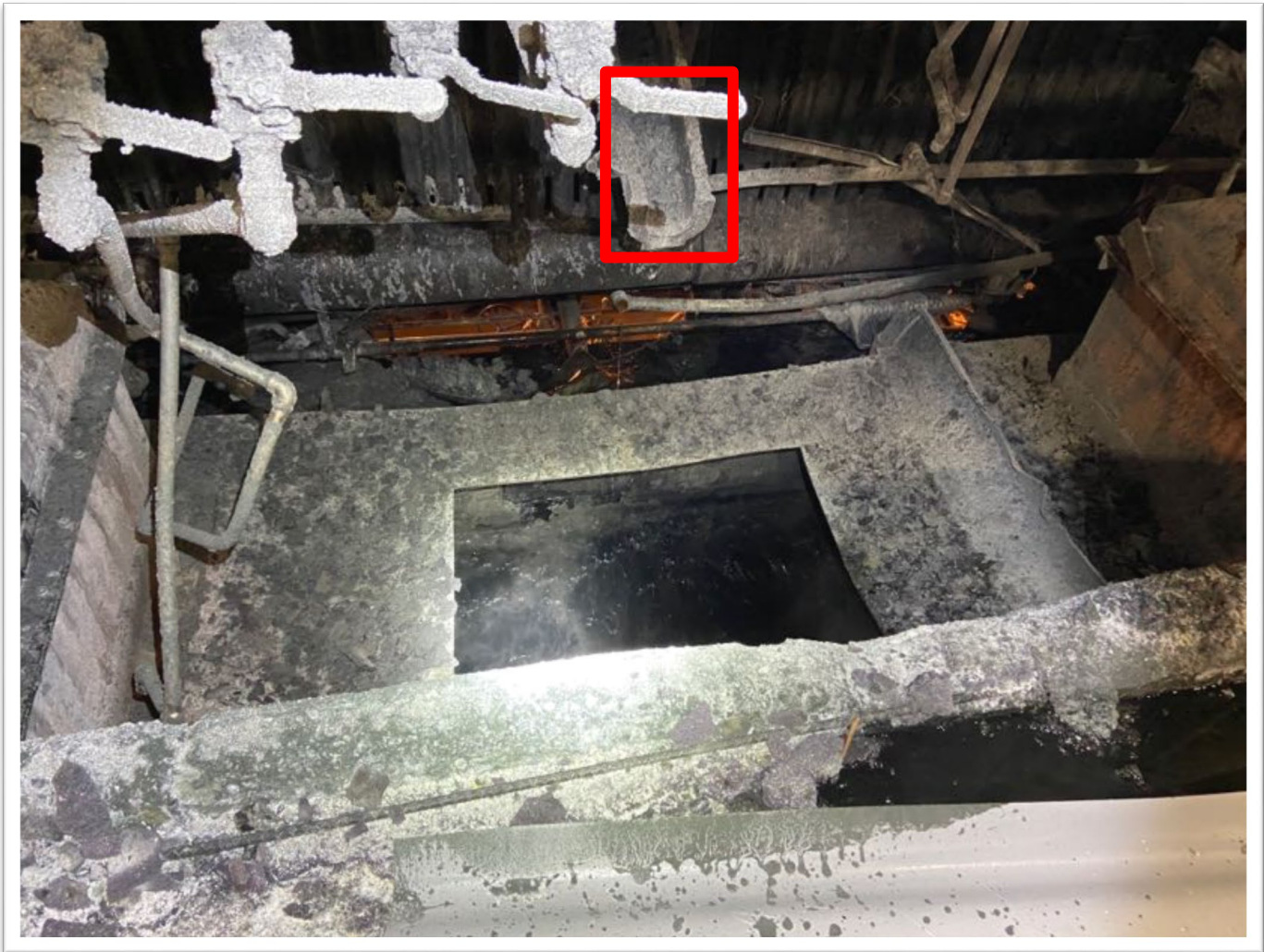
Photo 2 – RED: Smelt spout and opening to dissolving tank. Note that the shatter spray cover is missing and was later found inside the tank.
