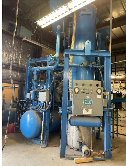
*Figure 4: P34 Skids Pre-Incident; high-pressure receiver and compressor on left; freezer and hand expansion valve on right*
