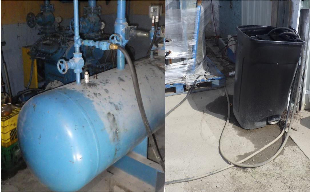
*Figure 13: Hose connected to the P24 high-pressure receiver (left) and piped into a garbage bin outside (right)*
