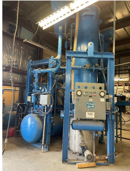
*Figure 4: P34 Skids Pre-Incident; high-pressure receiver and compressor on left; freezer and hand expansion valve on right*
