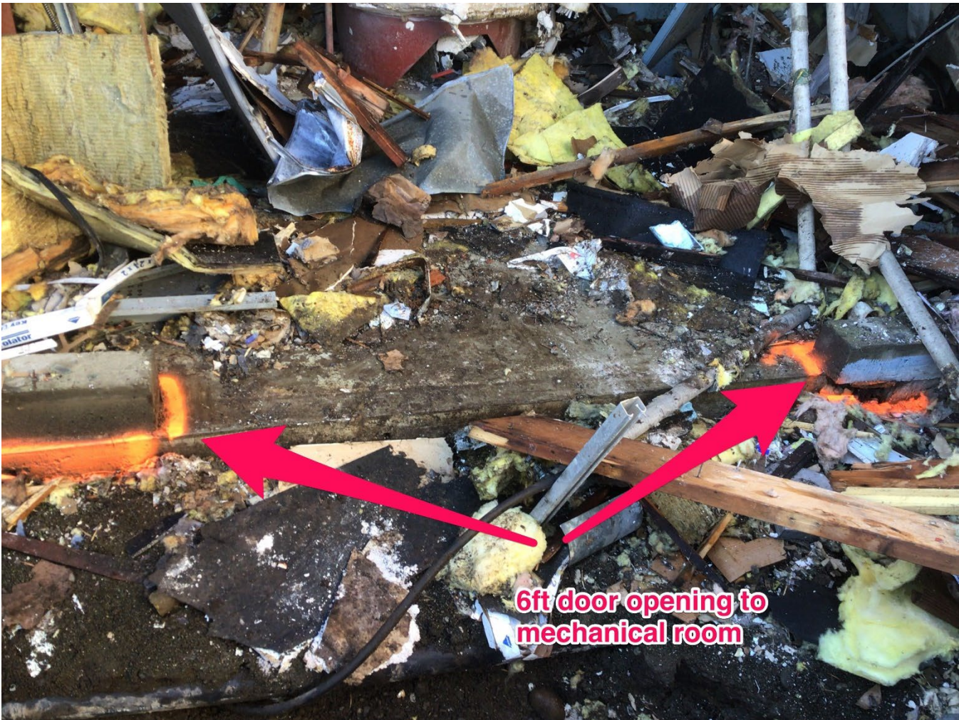
Image 8 -Opening to mechanical room with orange paint marking the edges of the doorway that was not installed at the time of the explosion.
