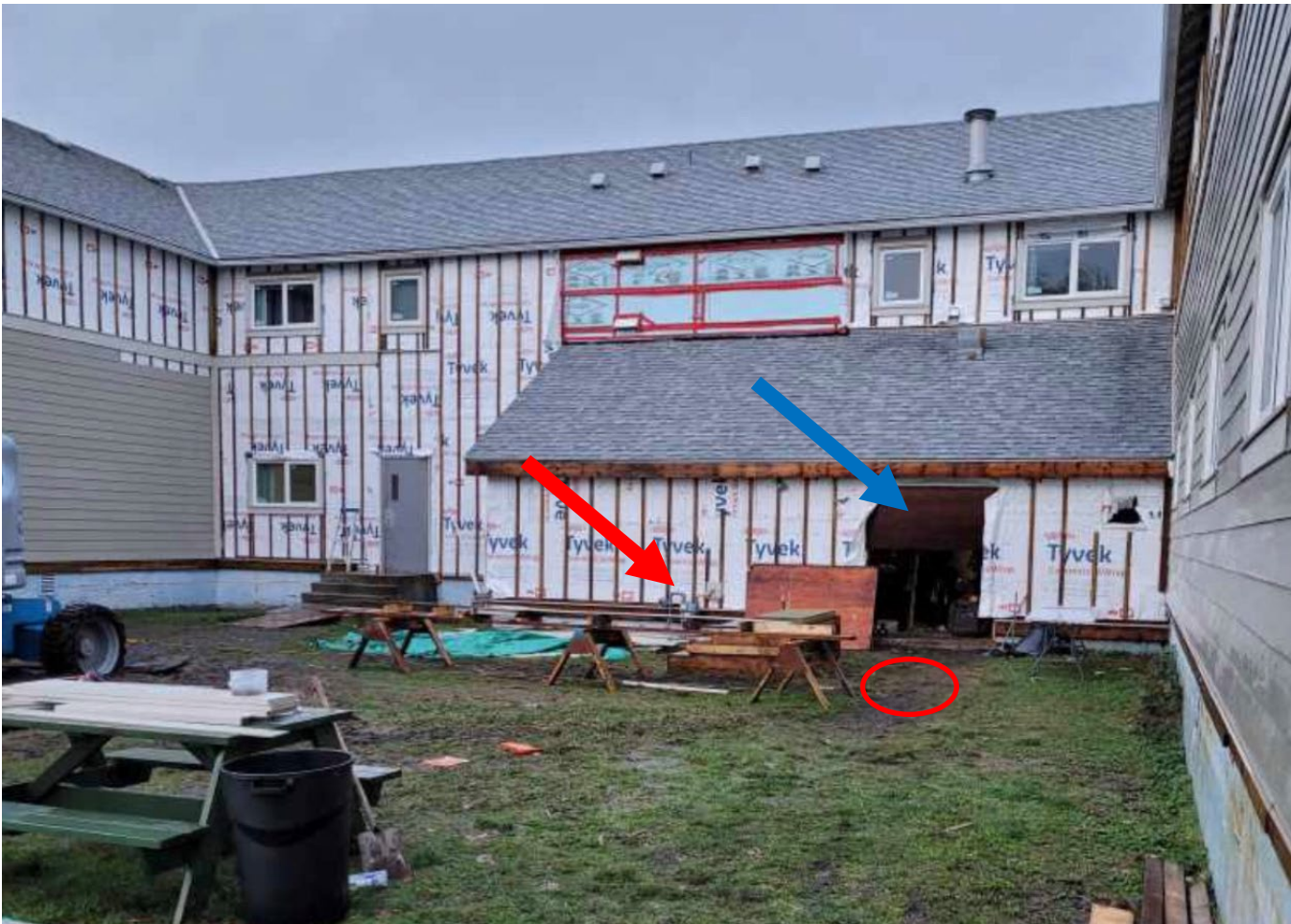
Image 1 – East side of building prior to incident. Red arrow indicates location of gas meter. Blue arrow indicates the mechanical room door opening with door removed. Red oval indicates location of gas pipe strike.
