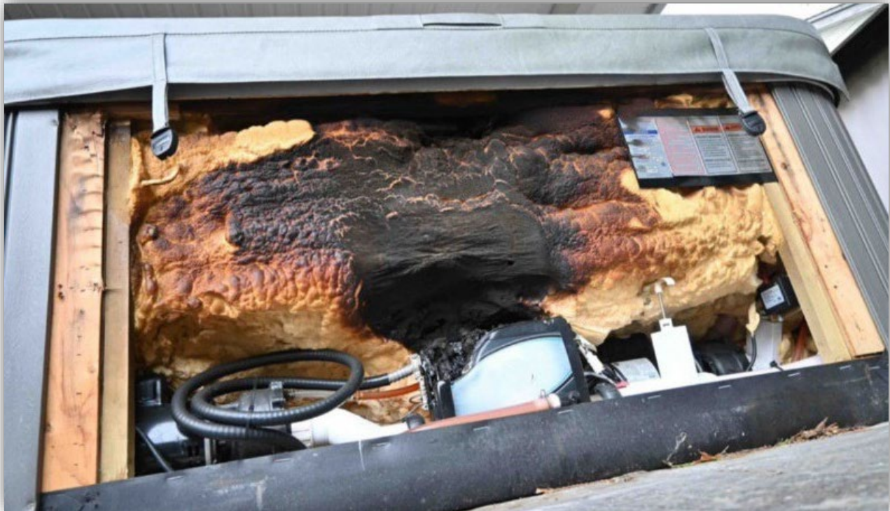
Image 3 – Close up of damaged hot tub.
