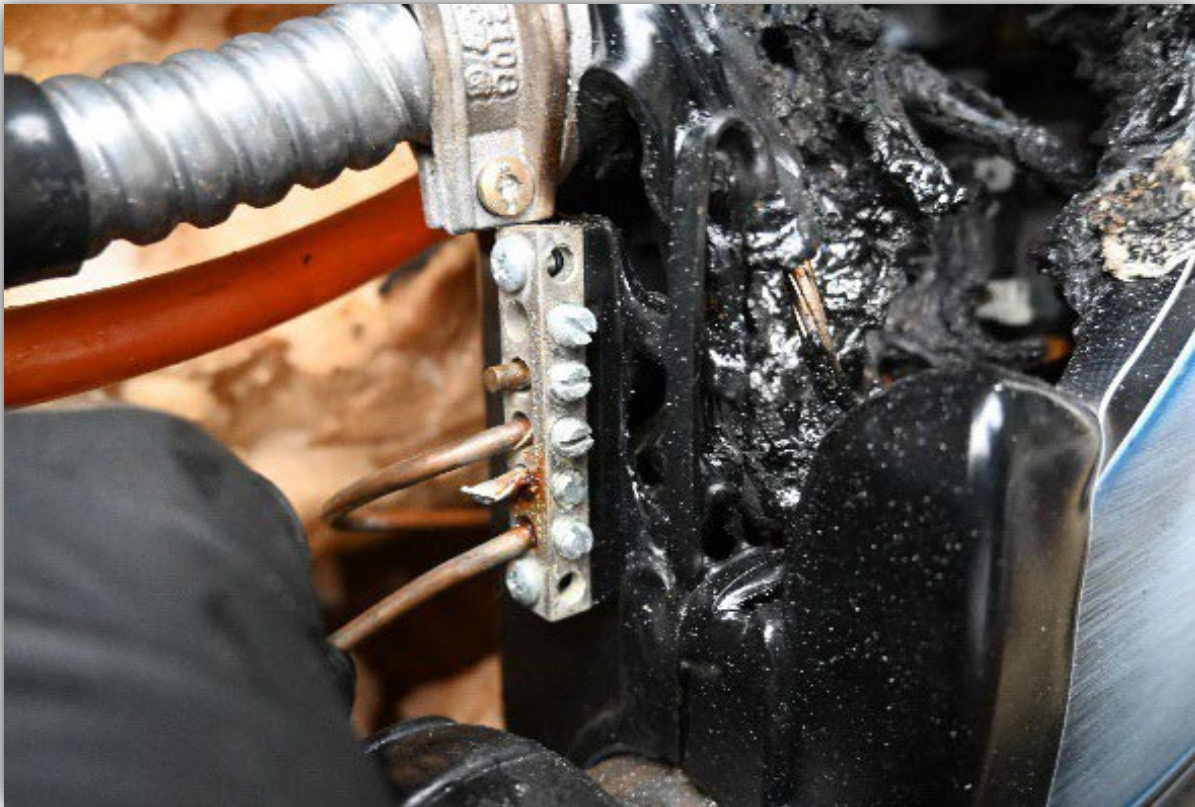
Image 2 - Aluminum cable installed to hot tub controller.
