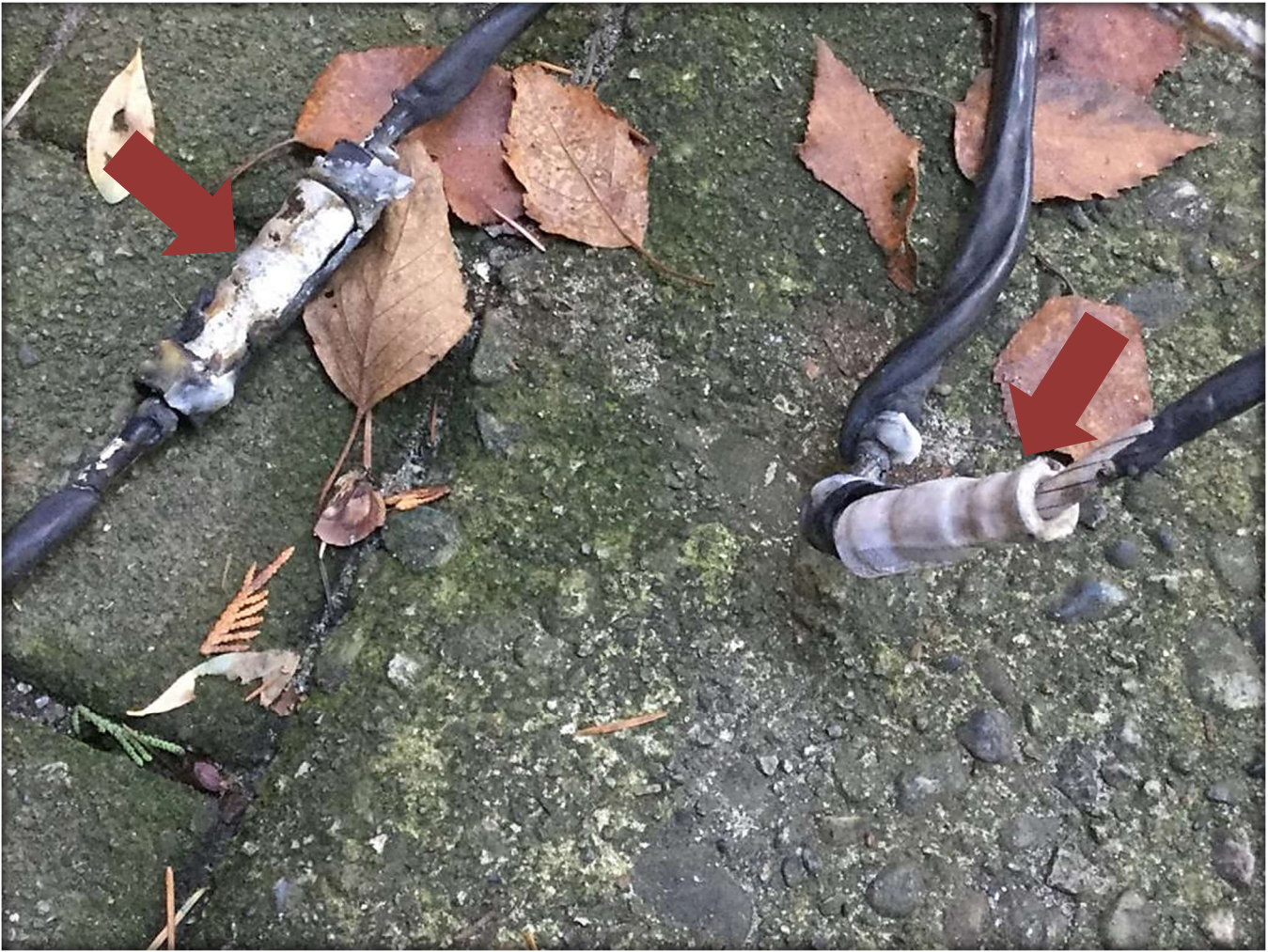
Figure 2 - 240 volt conductor compression connectors without insulation (arrows).
