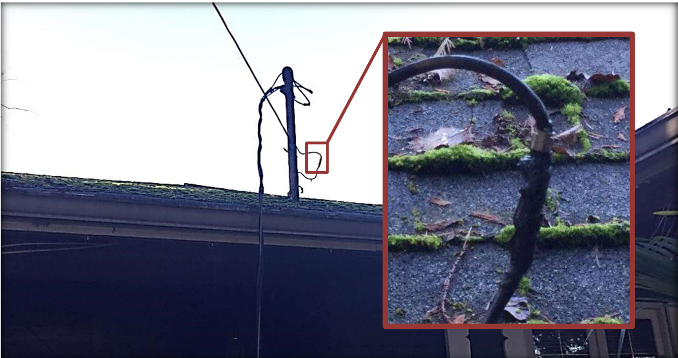
Figure 5 - Closeup of cable TV service drop splice with melted tape.
