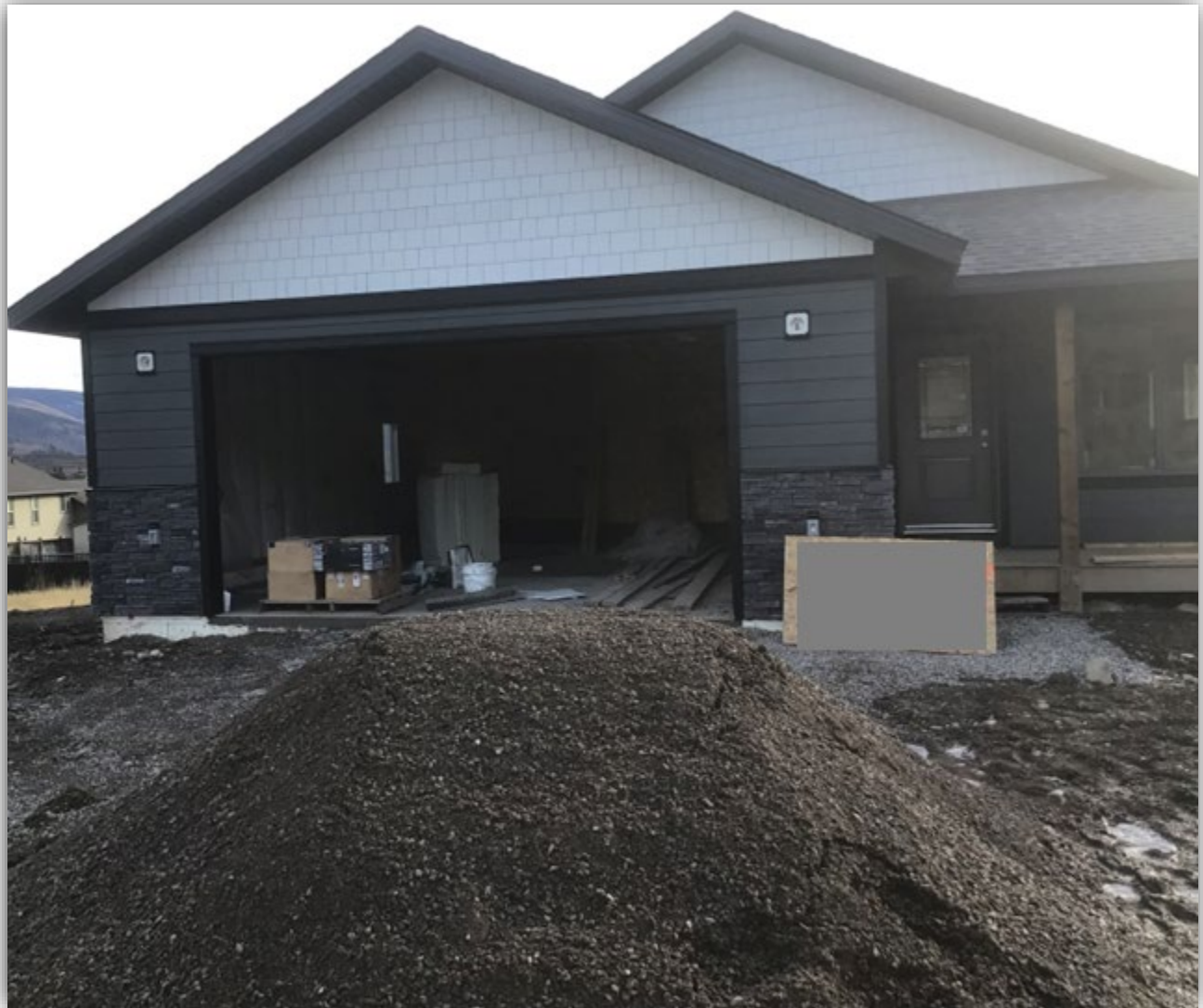
Image 1 – Front of house under construction.
