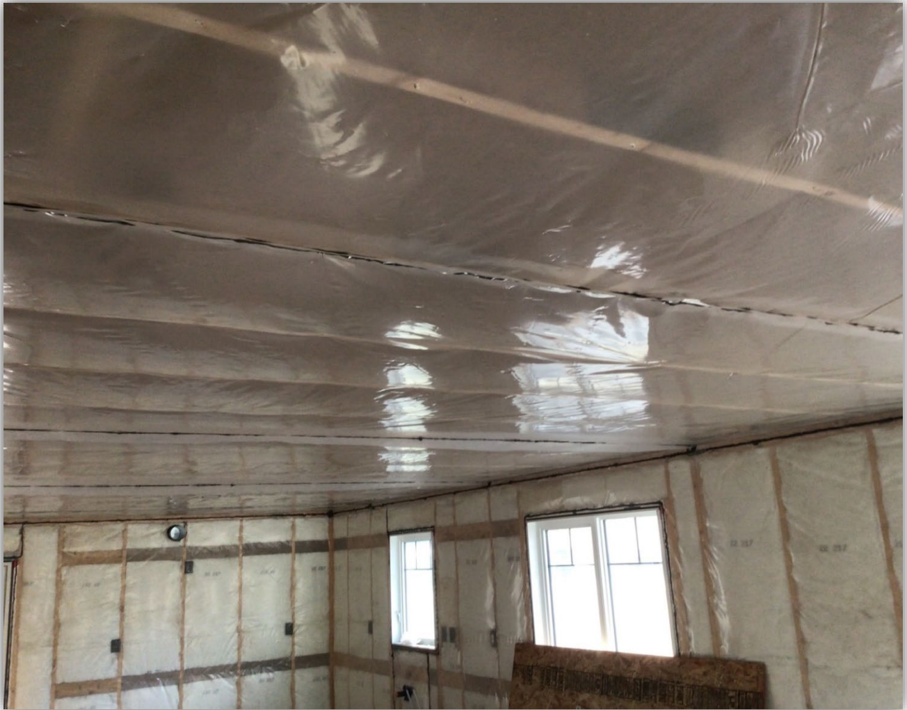
Image 4 – Fiberglass insulation and vapor barrier showing home sealed from fresh air.
