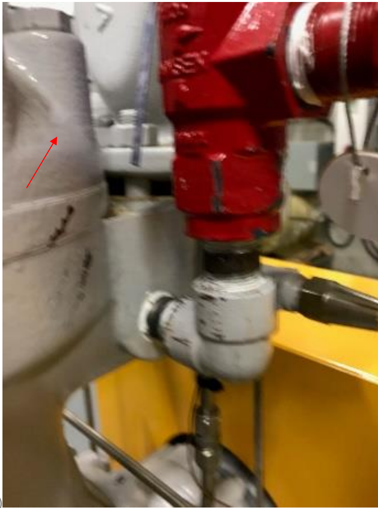
Normal Pipe Size \frac{3}{4} close nipple upstream of elbow.
