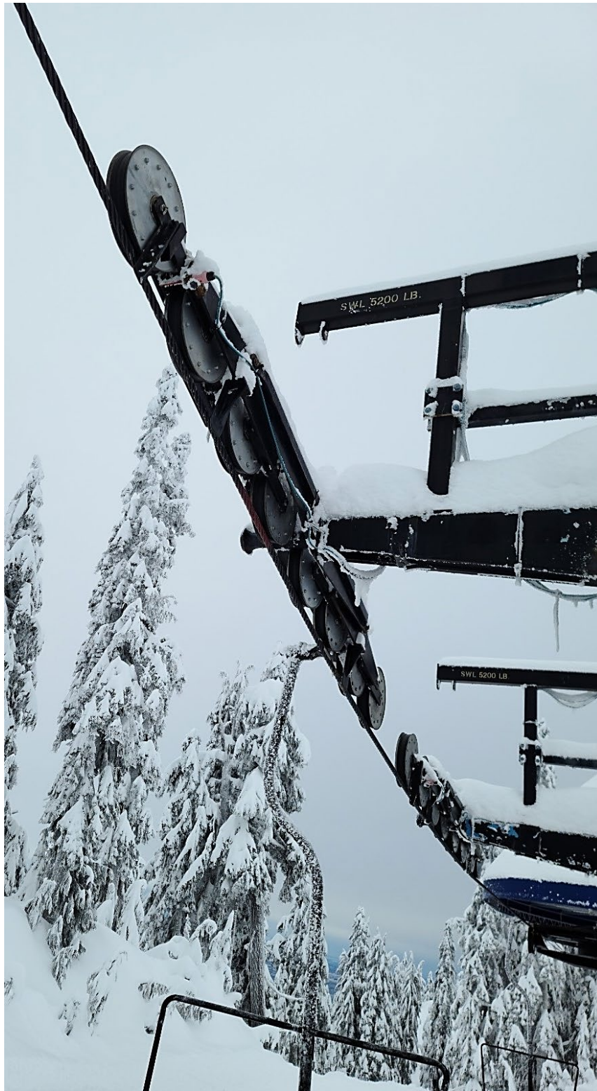
Photo 5 - Tower 2 downhill side where the unloaded carrier with the partially attached grip, contacted the compression sheave assembly, and fell to the snow.
