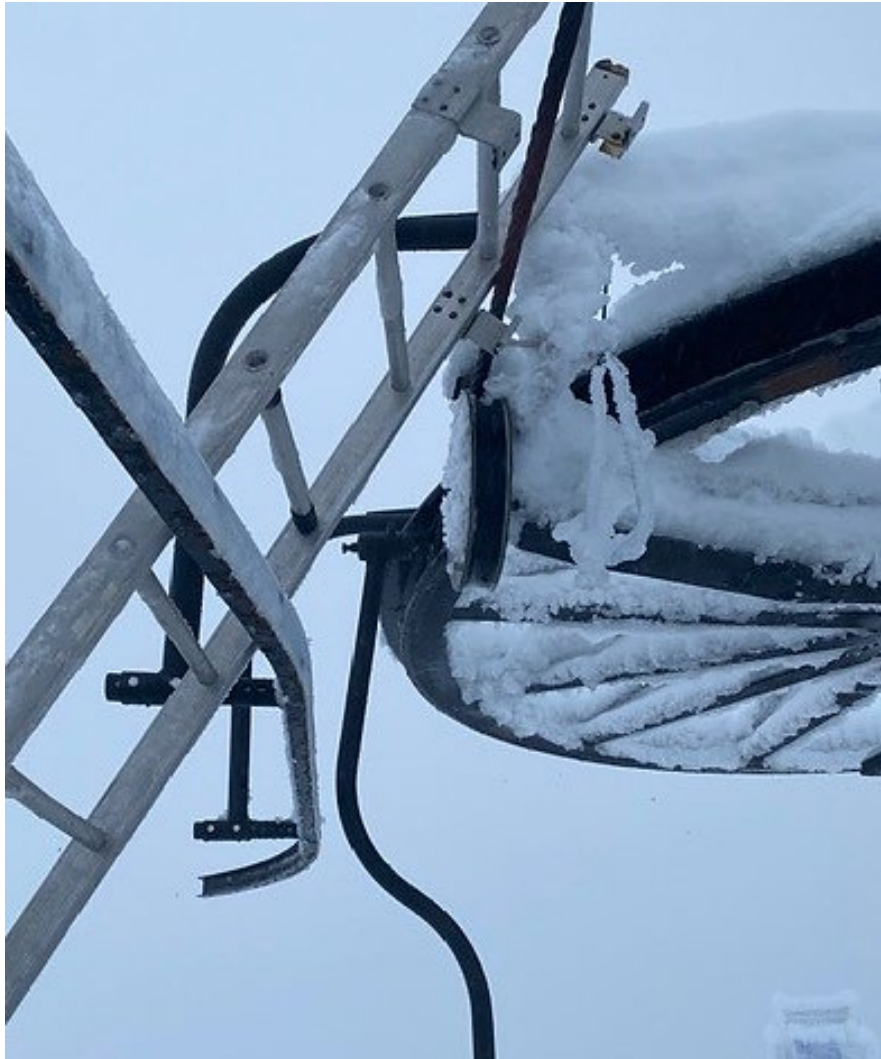
Photo 3 - Chair guide located at the top terminal, controls chair swing as the grip enters the bullwheel.
