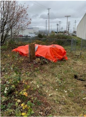
(Photo #3) east pole
