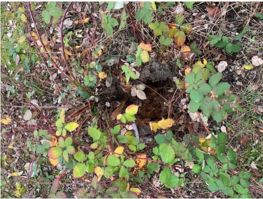
(Photo #4) west pole base in soil
