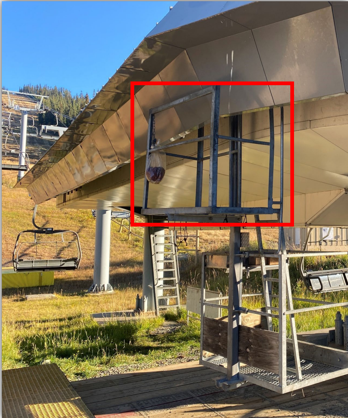
Photo 4 – A different work carrier at another lift at the same facility. [RED] Fixed upper platform handrail that clears the station without the need to be lowered.
