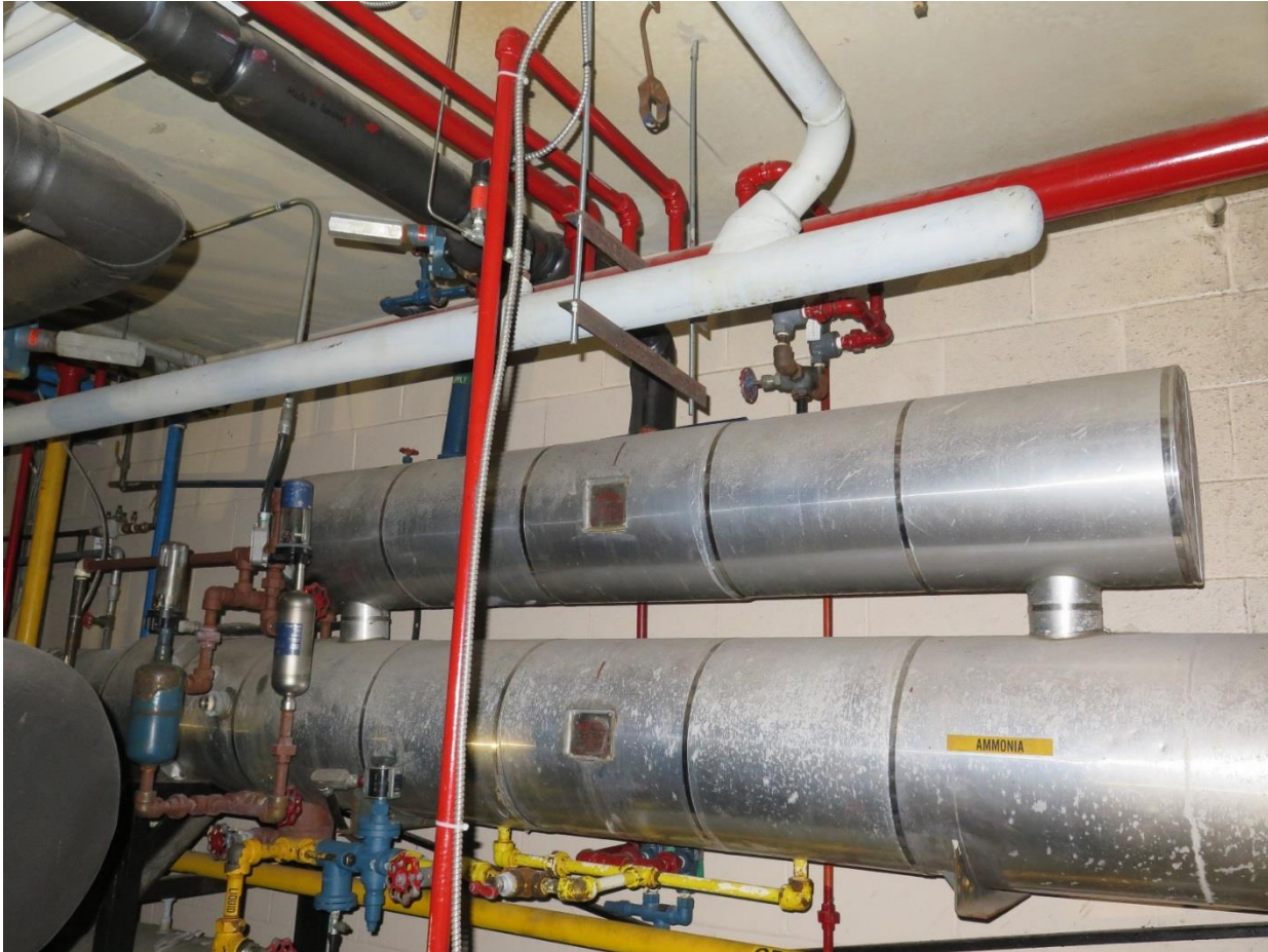
Photo C3-12: Curling chiller (with insulation) showing the ammonia liquid inlet configuration. Valve positions are noted in Appendix B.
