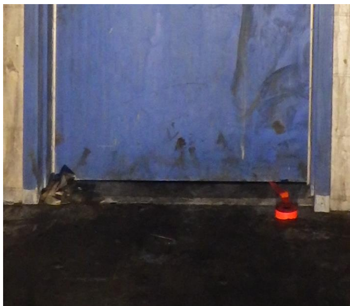
Photo C6-10: Door between mechanical room and vestibule showing gap under door.
