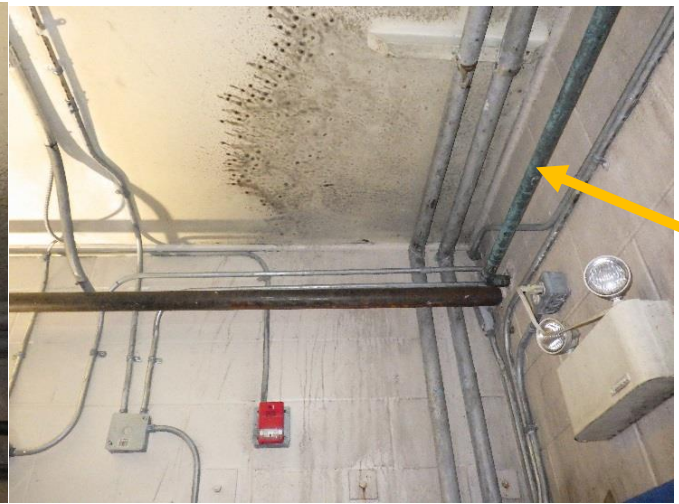
Photo C6-2: SW corner of the mechanical room (above the door to vestibule). Brine spray is seen on the ceiling and walls below. The arrow indicates blue/turquoise discolouration on the copper pipe from exposure to ammonia.
