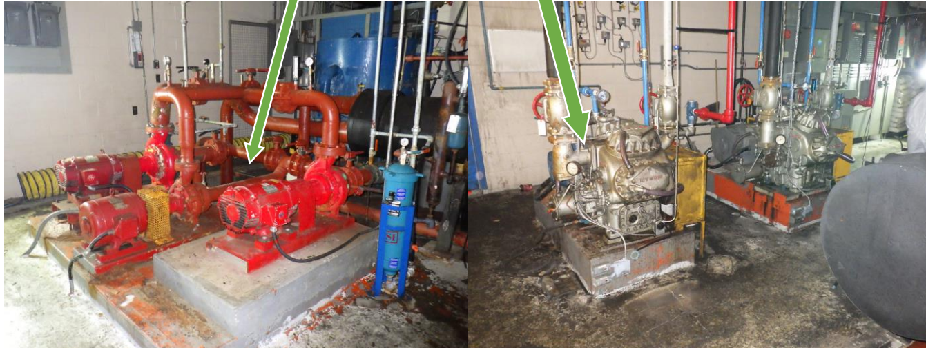
Photo C2-2: Arena pump, standby pump, curling pump. These pumps are visible in the background of photo C2-1.
