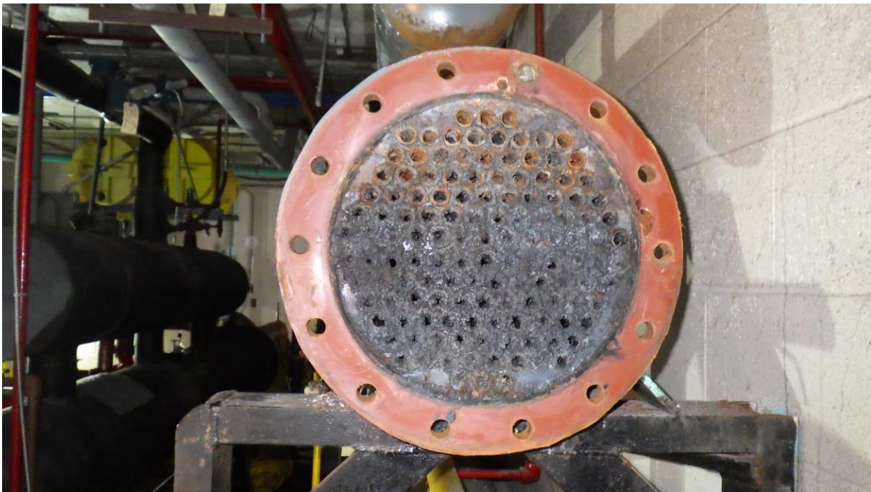
Photo C3-4: Curling chiller, tube sheet upon opening in January 2018 showing residue.
