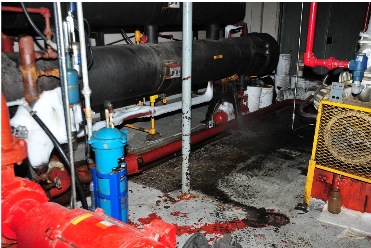
Photo C6-9: Projected contents of the brine piping from the separating coupling.
