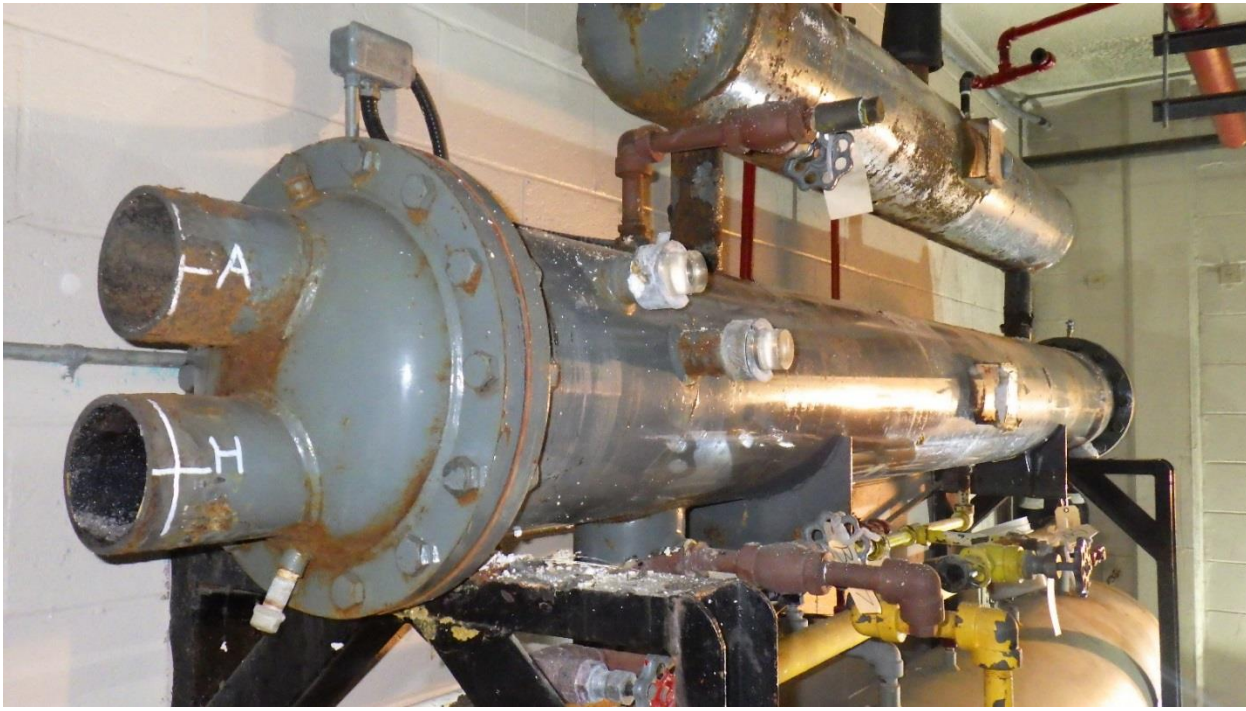
Photo C3-1: Curling chiller with the brine inlet and outlet piping removed. The photo below shows the curling chiller with its head removed, exposing the tube sheet.
