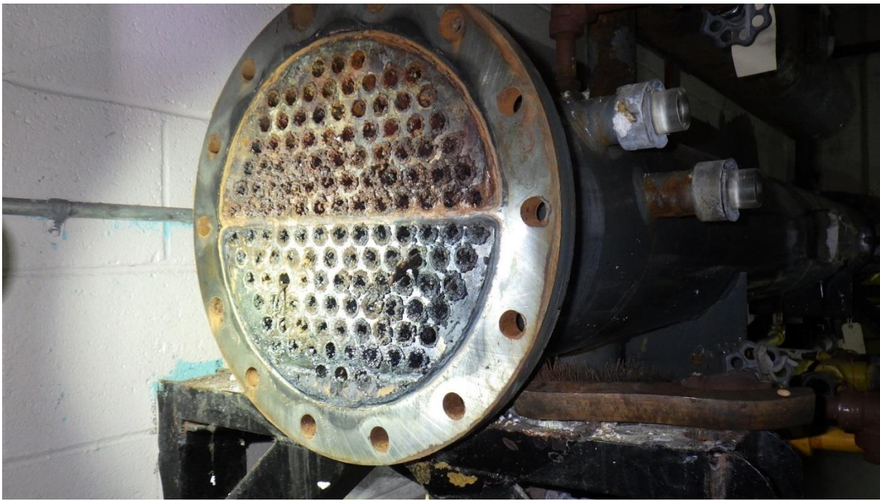
Photo C3-2: Curling chiller, head removed. The brine inlet/outlet tube sheet at the north end of the chiller. Debris and residue is visible on the tubes.
