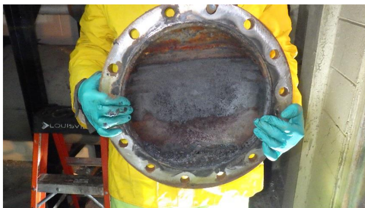
Photo C3-5: Close up of upper tubes from return end of chiller upon opening in January 2018.
