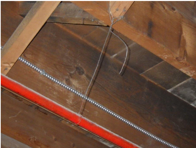
Photo C7-2: Close up of the emergency discharge piping from the mechanical room into the figure skating storage room. The photo shows a costume suspended from the piping.
