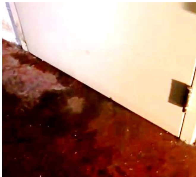
Photo C6-11: Door between vestibule and arena did not incorporate a seal at bottom.
