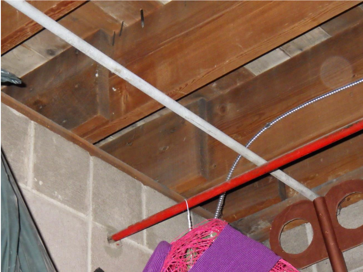
Photo C7-2: Close up of the emergency discharge piping from the mechanical room into the figure skating storage room. The photo shows a costume suspended from the piping.
