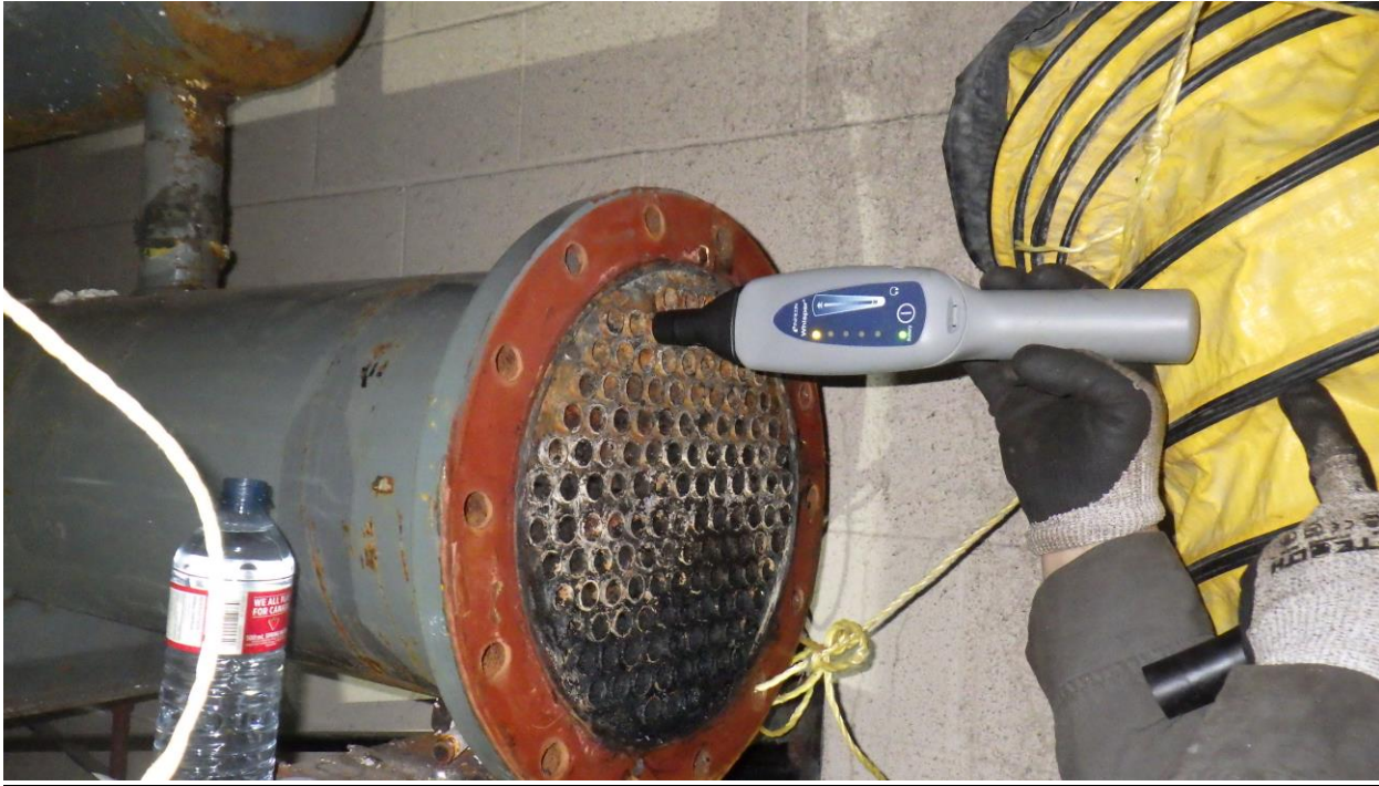
Photo C3-3: Return end tube sheet (south end) of the curling chiller. Debris and residue is also visible on the tubes and sheet.
