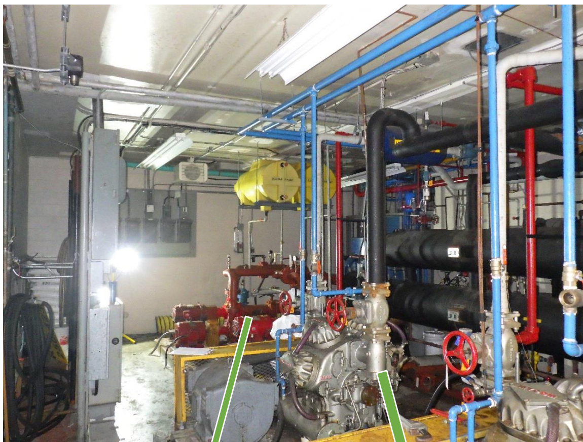
Photo C2-1: View looking from corner with vestibule door showing compressors in the foreground, expansion tanks near the ceiling and the black insulation covering the arena brine system chiller and surge vessel.
