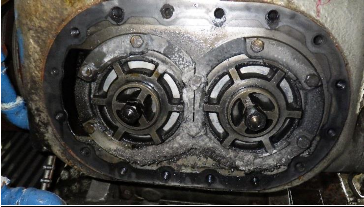
Photo C4-3: Close up of the lower valves in photo C4-2. Build-up of salt crystals from brine around the valves compressors #1 and #2.
