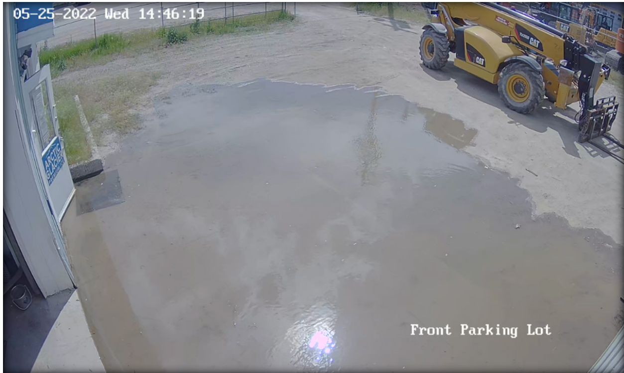
Figure 2 - Flooded parking lot from the “purging” of the P24 system
