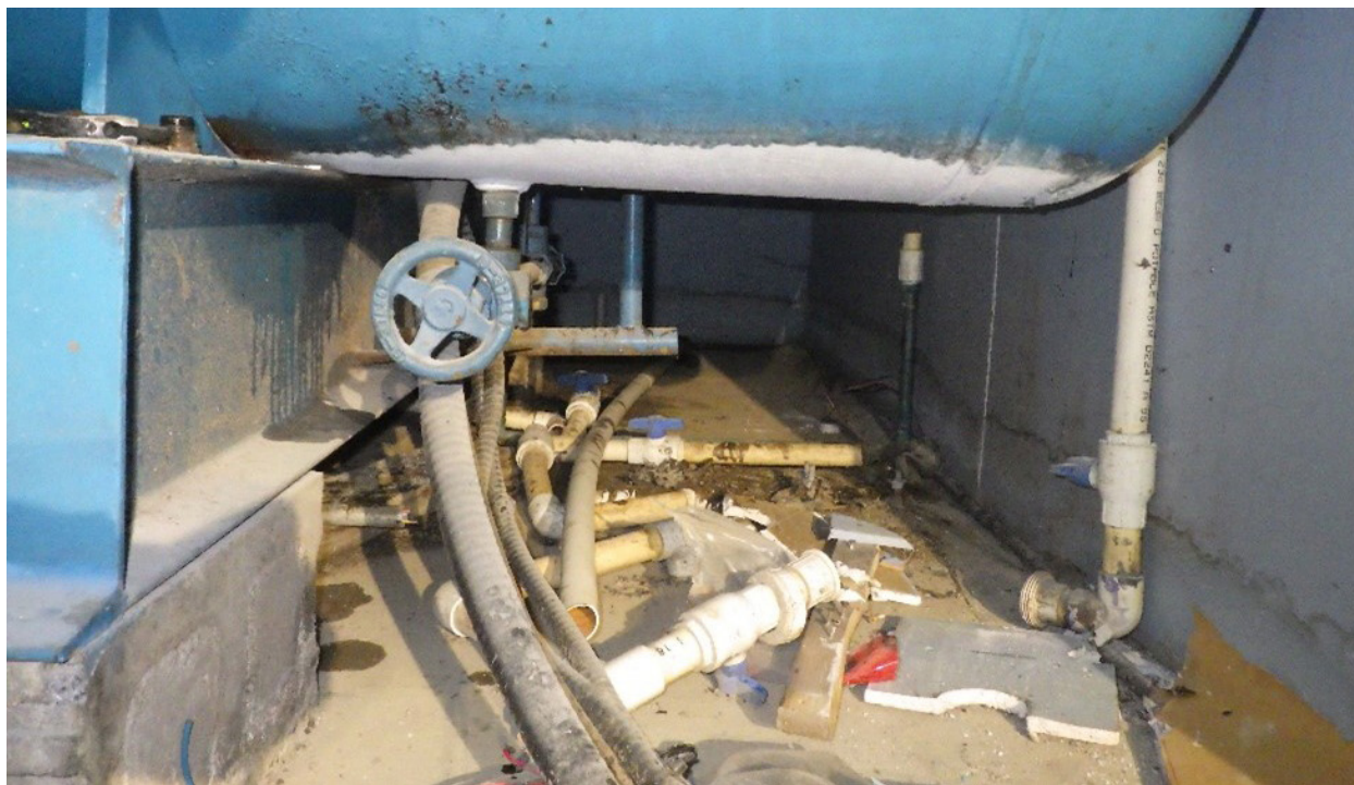
Figure 3 - Distinct frost line showing liquid ammonia levels in the P24 system during purging by Technical Safety BC post-incident..
