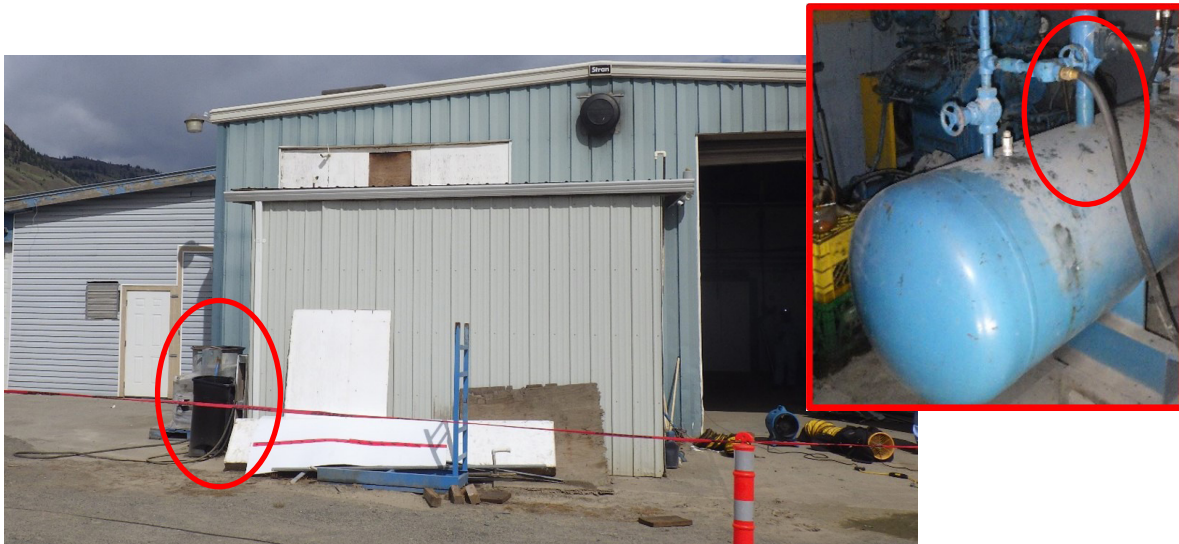
Image #2 - Purge vessel and hoses that were in place prior to the incident. Hoses were connected to a water source and the ammonia receiver (red square) in the side building.
