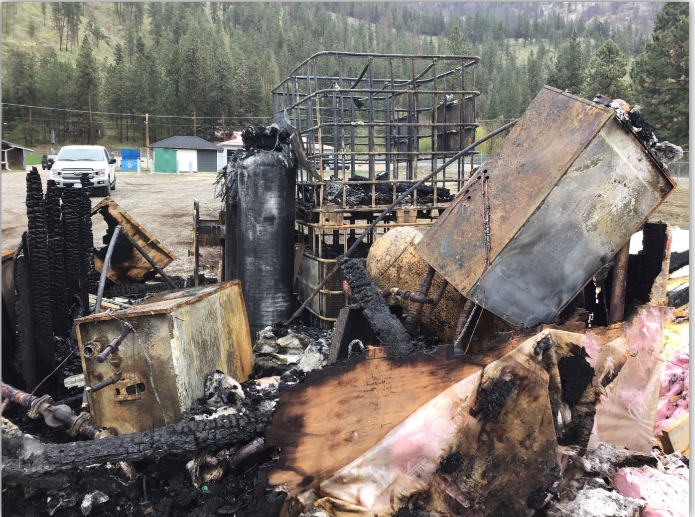
Image 17 – View of Mechanical room from south side, evidence of structure plywood and insulation not fully destroyed. Boiler noted at upper-right of photo. Metal water racks still standing, plastic interior water containers destroyed.
