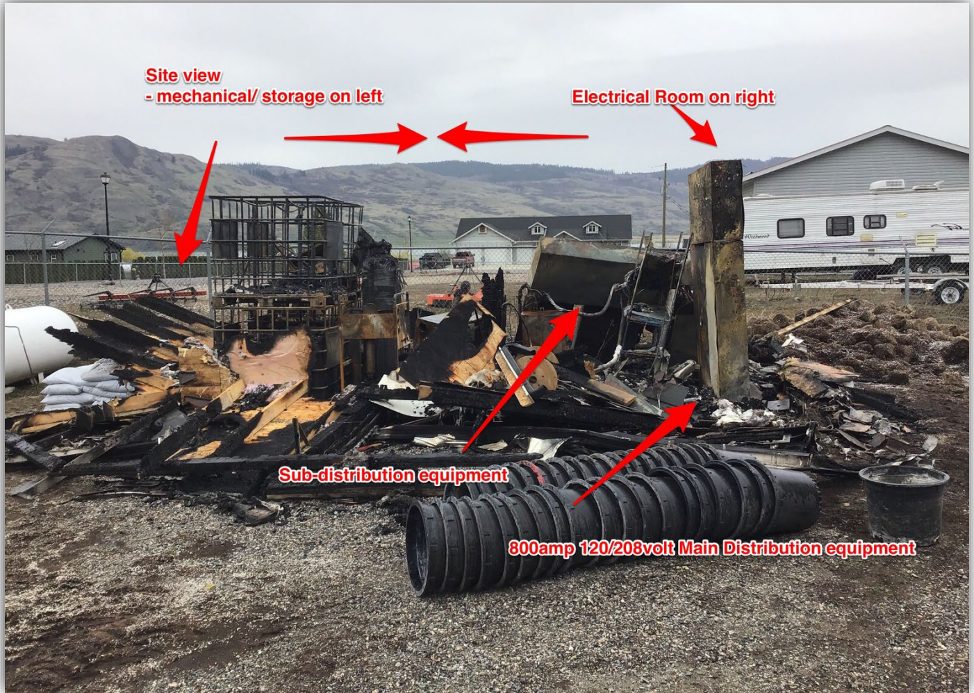
Image 2 – Site view facing south of as-found site review.
