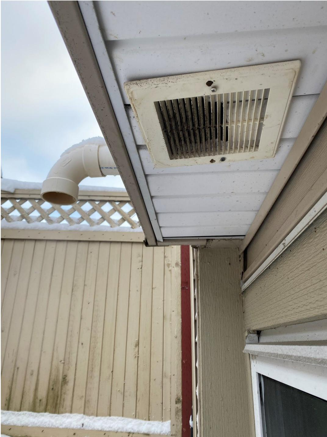
**Photo 11** - The ventilation opening for the gas fireplace cavity that flue gas containing 168ppm of CO was measured migrating into the home.
