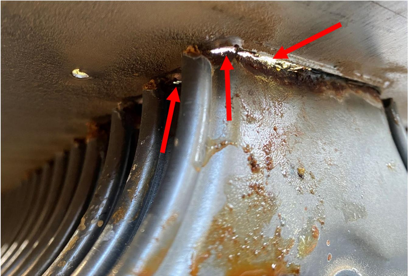
**Photo 5** – Red arrows show light passing through holes from corrosion where the tube connects to the coupling box from the exterior.
