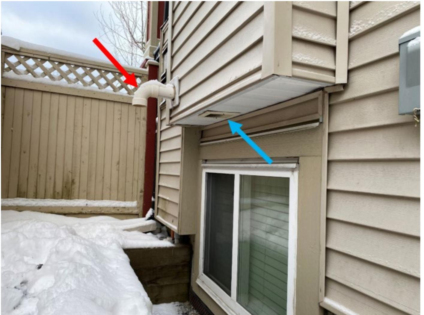
**Photo 10** – **Red** shows furnace vent termination with a 90-degree elbow pointing down. **Blue** shows ventilation air opening for gas fireplace cavity.
