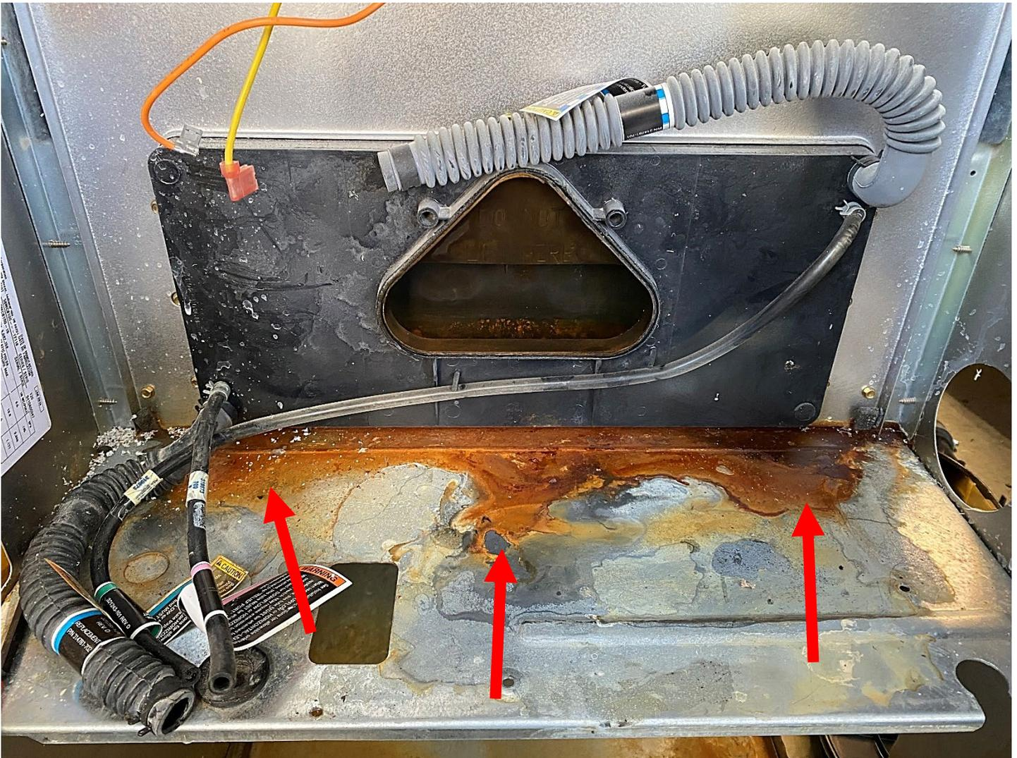
**Photo 3** – Red arrows show areas of the furnace case stained and corroded from condensate leakage.
