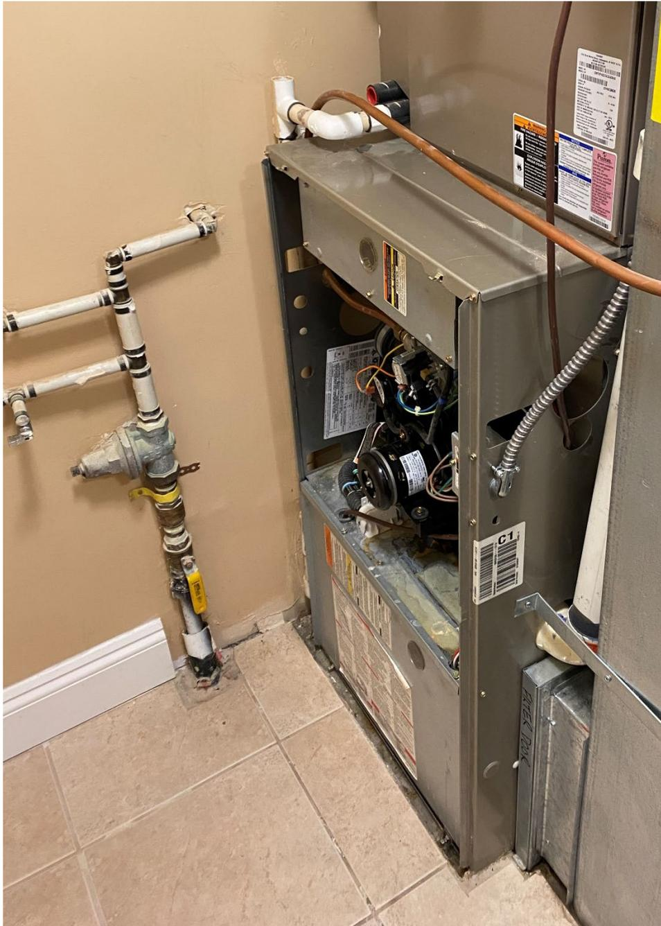
**Photo 1** – Furnace installed in basement of home in the up-flow position
