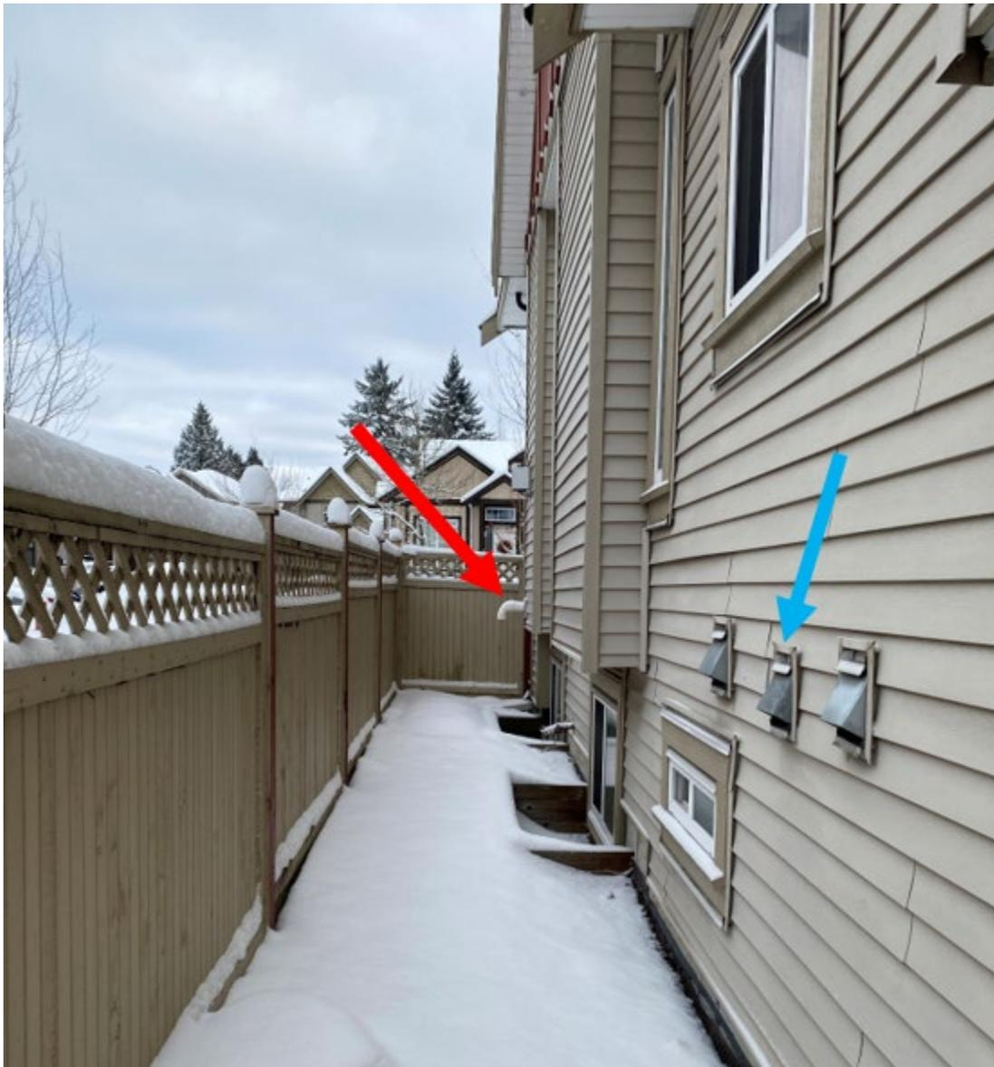
**Photo 9** – **Red** shows furnace vent termination at side of house. **Blue** shows air intake grills to the house 24 feet away where flue gas containing 90ppm CO was measured migrating into the home.
