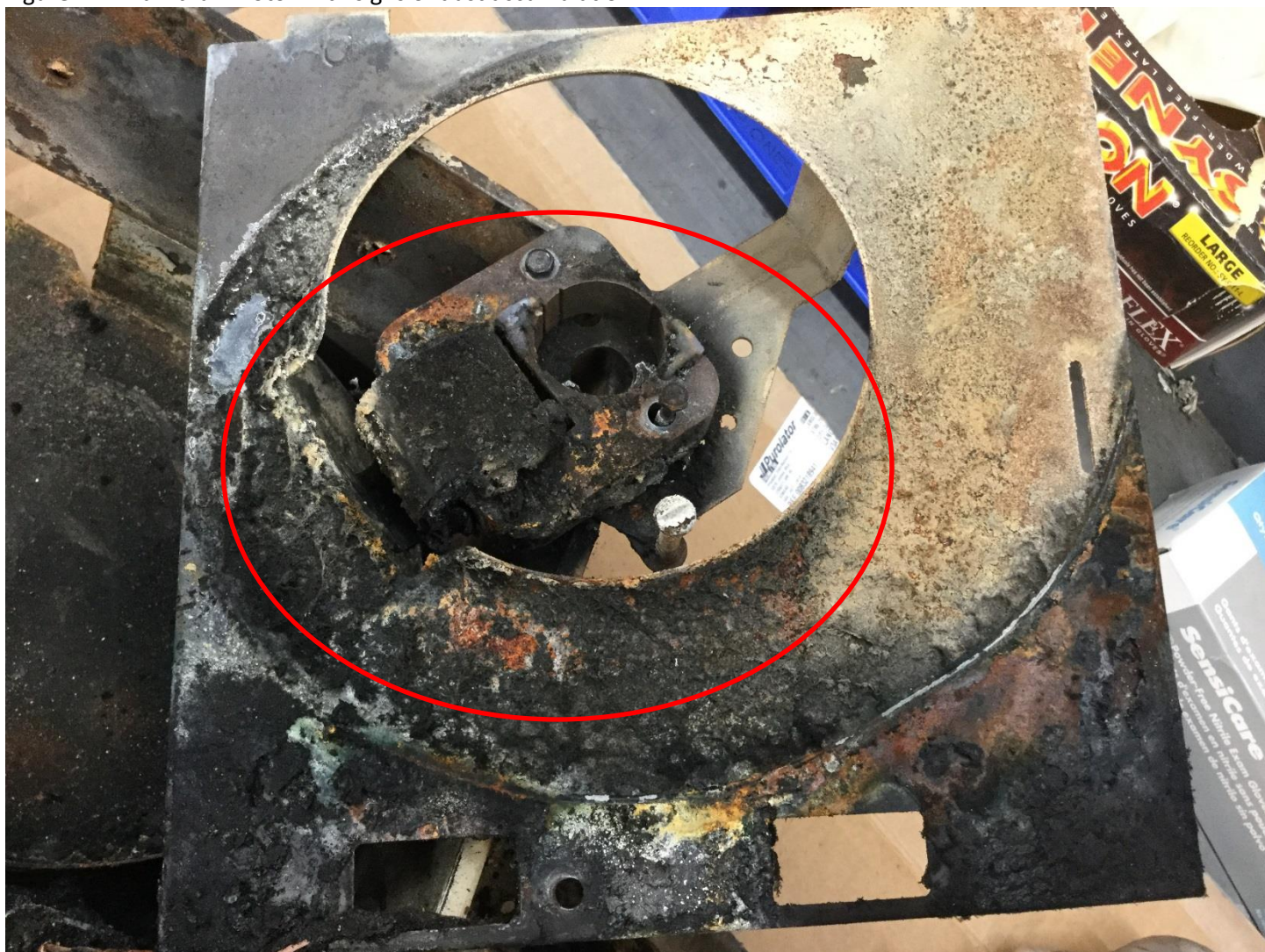
Figure #2 – Burnt fan motor with signs of dust accumulation
