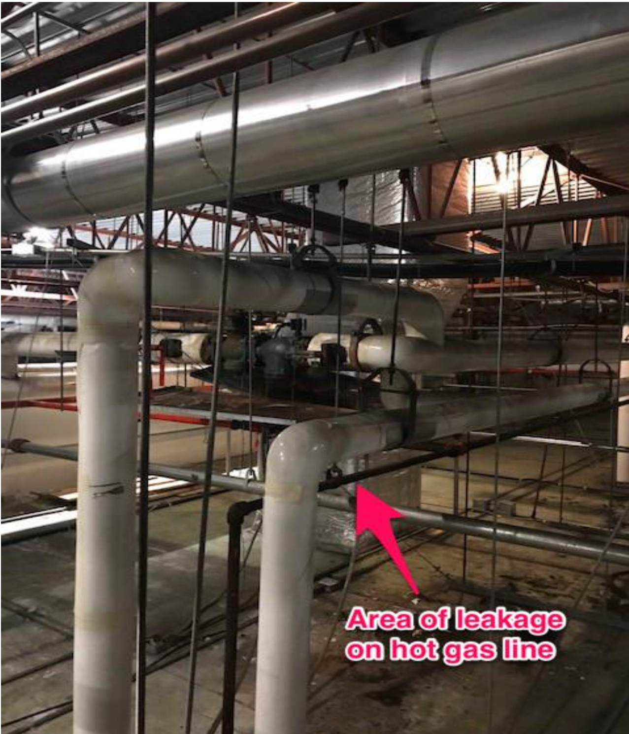
Picture 1 Mezzanine area above grinding room
