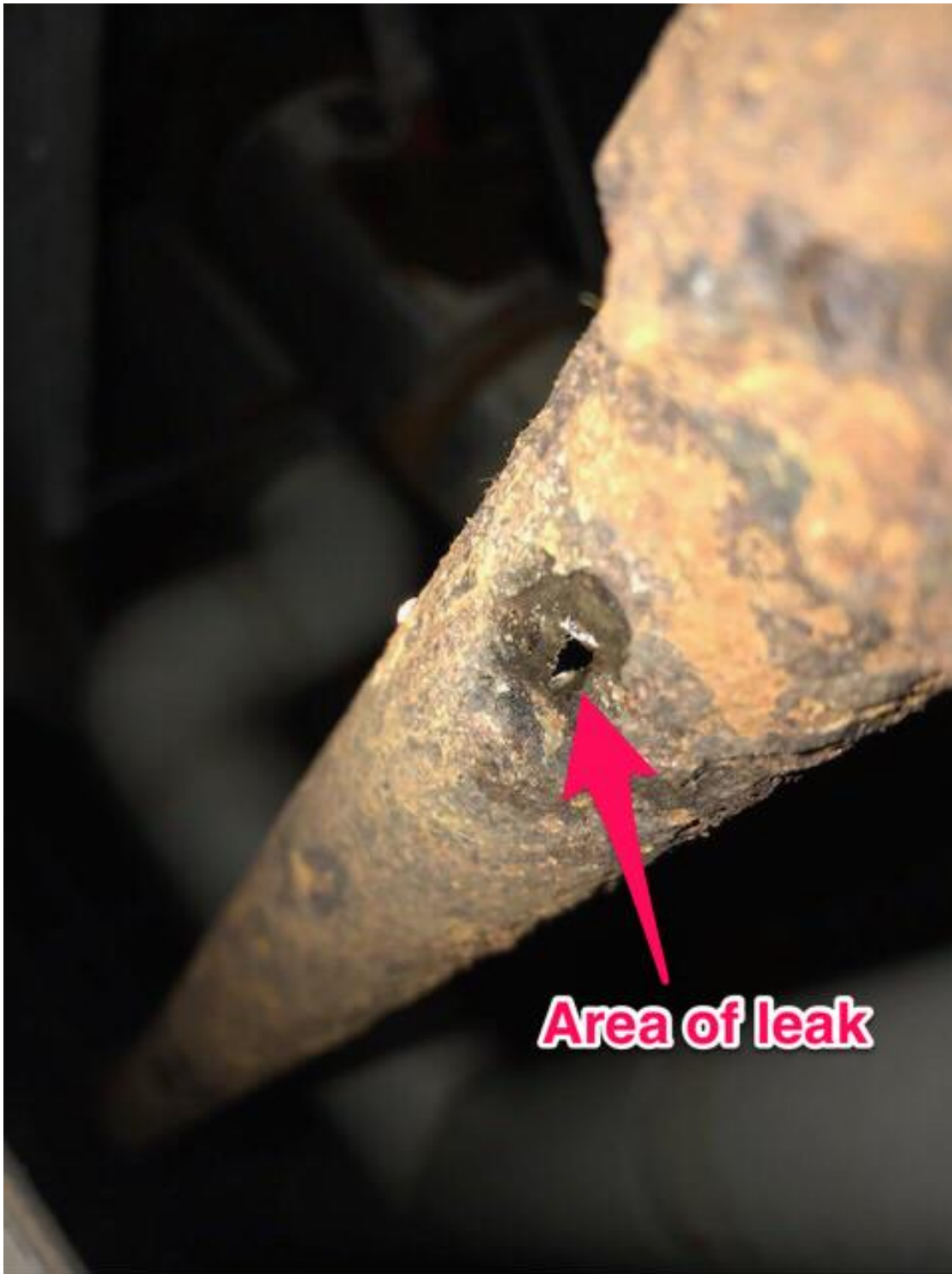
Picture 4 Close up of pin hole
