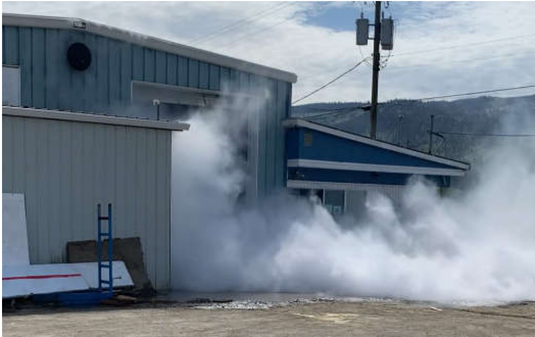
Figure 5: Ammonia cloud indicating a flashing liquid release.
