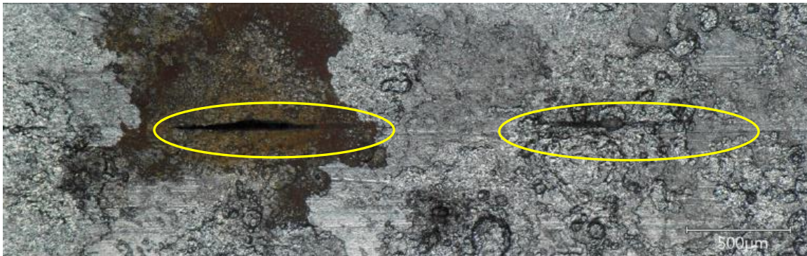
Figure 5: Cracks along the weld line on the outside wall of the tube.
