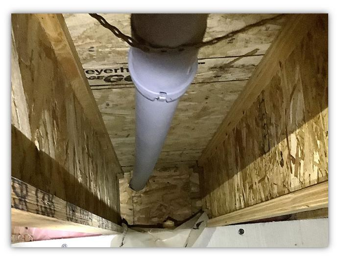
Image 3 – Exhaust venting to exterior.
