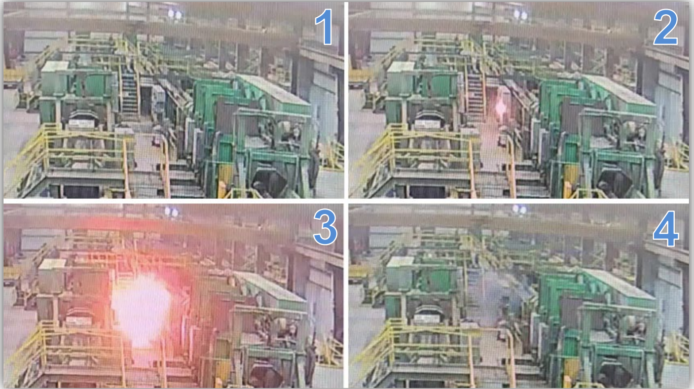
Image 6 – Screenshots of arc incident from the surveillance camera.
