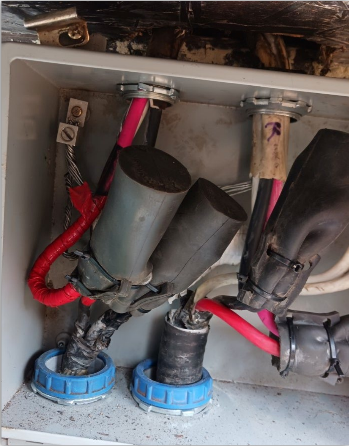
Image 4 – Junction box replaced, conductors re-terminated, re-insulated.
