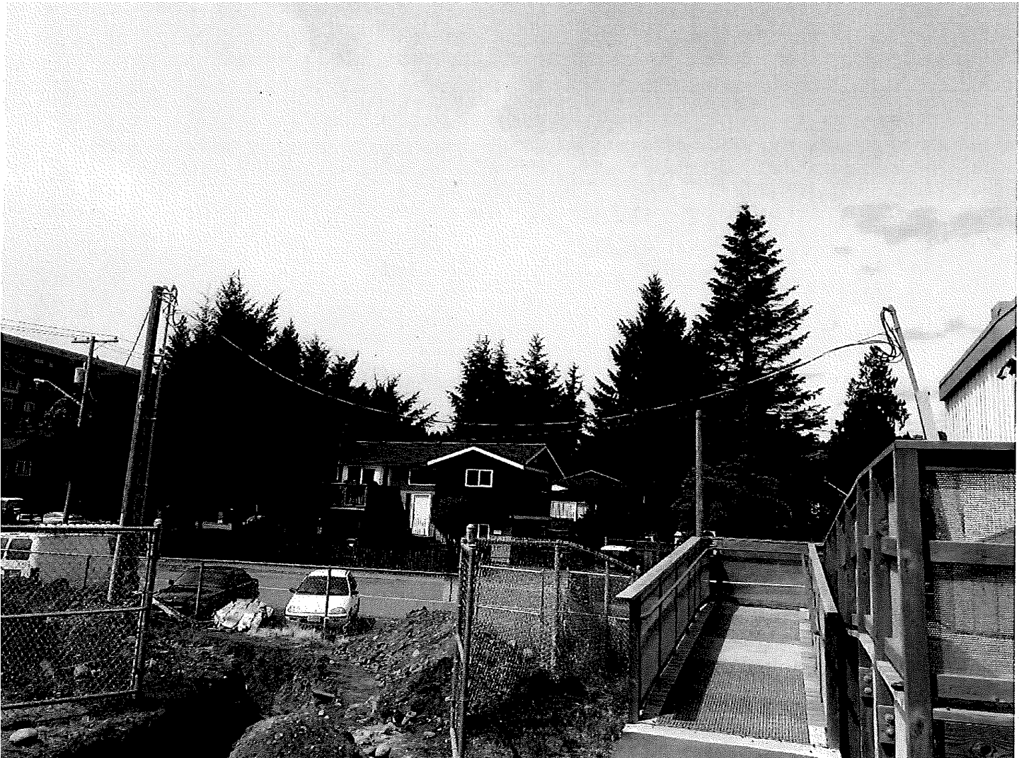
Photo 1: View of the suspended overhead electrical cable and bent vertical mast (right). Photo shows the equipment after partial repairs had been conducted, (provided by FSR).
