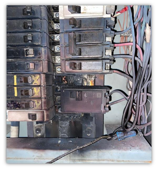
Image 1 – Panel showing damage from the short circuit.
