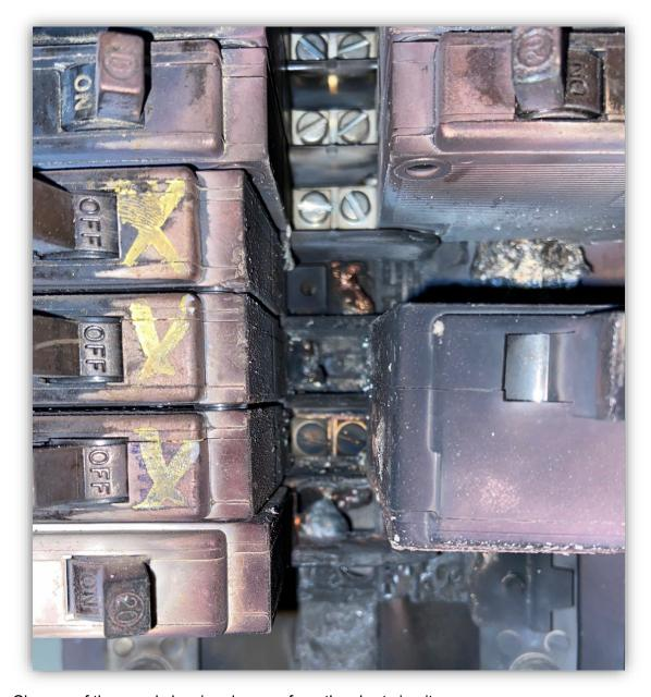
Image 2 – Closeup of the panel showing damage from the short circuit.
