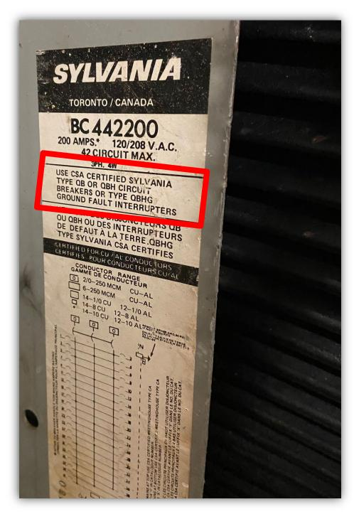
Image 3 – Panel schedule showing compatible breaker types.
