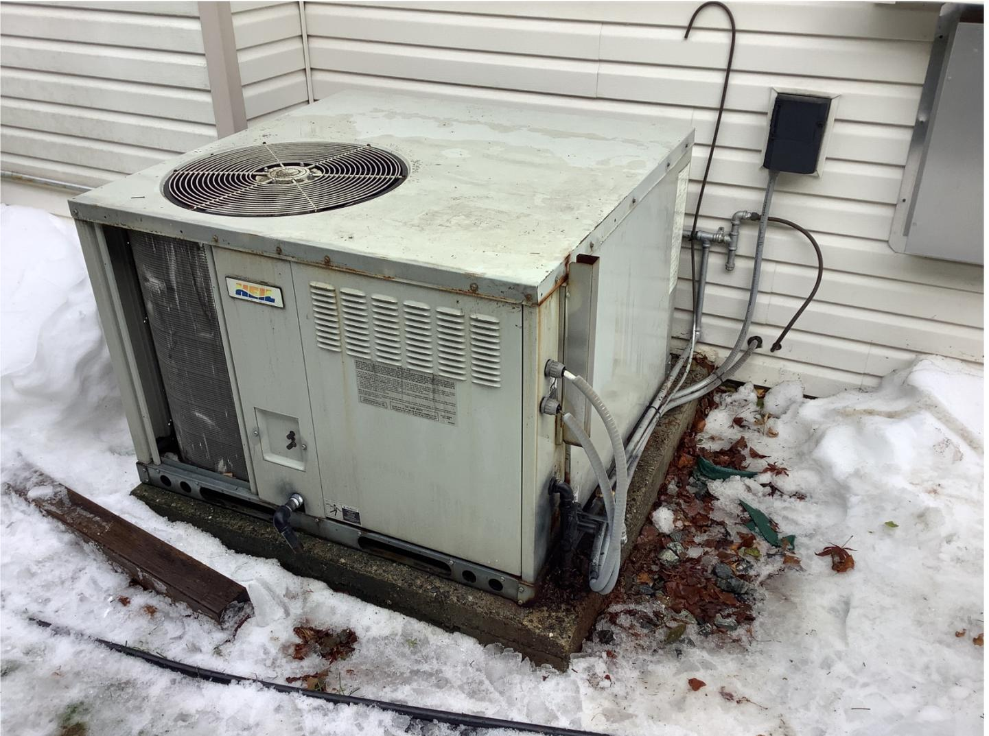
Image 2 - Outdoor heating unit pictured above. Supply and return duct connections cannot be seen in the picture but are located below the unit and ducted down through the concrete pad and into the crawlspace where they are connected to rooms in the home.
