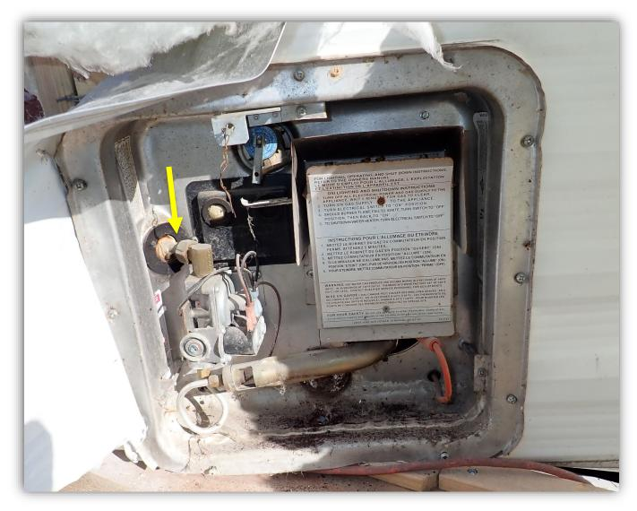
Image 7 - Interior of trailer water heater showing piping configuration. Arrow indicates propane supply piping.
