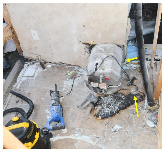
Image 10 - View of bathroom at time of investigation. Arrows indicate area where copper propane tubing left floor and connected to water heater. Note burn marks around where propane tubing left floor.
