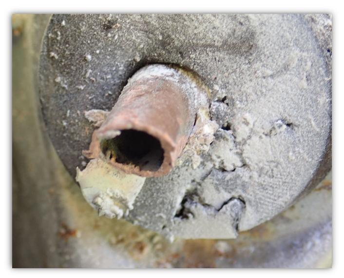
Image 11 - Close up of cut copper propane tubing.
