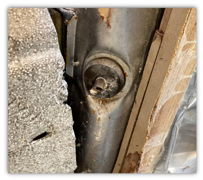
Image 9 - Alternate view of propane tubing connection to water heater.
