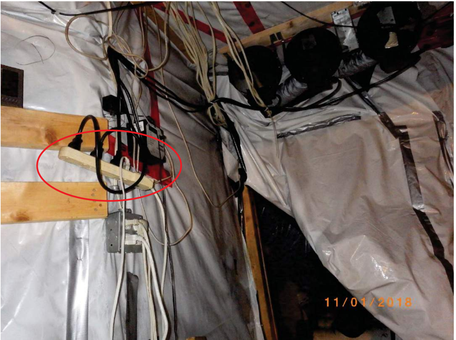
Figure 8 – This photo shows an exemplar power bar (red oval) used in another part of the basement area. Both figures 7 and 8 show that the power bars were similarly used throughout the basement. These configurations and use are similar to the configuration at the point of origin.
