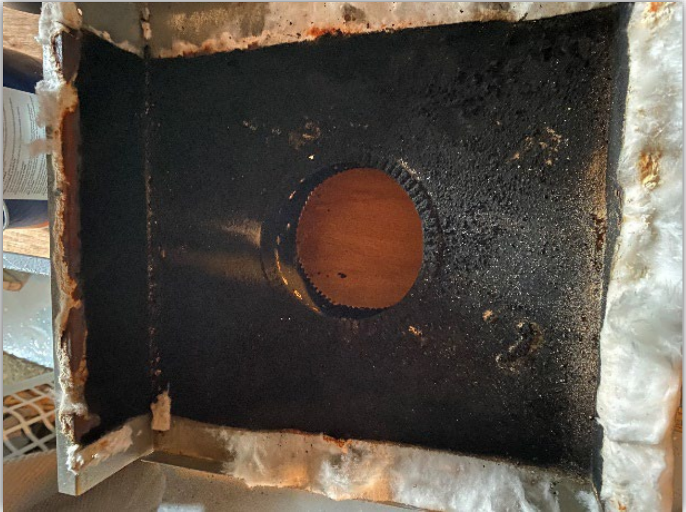
Image 3 - Top cover of the heat exchanger. This will seal in the burner compartment from the outside of the boiler and convey flue gases through the centre hole to flue.
