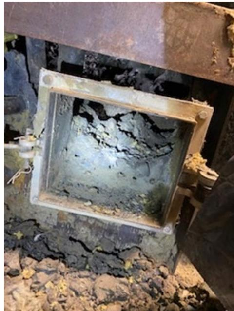
**Outer shell steel melted away.**
