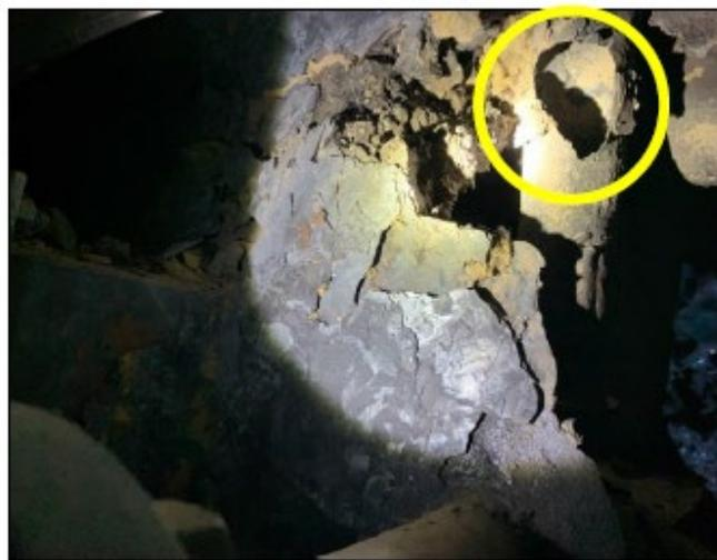
**Failed shell and hole in soot blower piping.**
