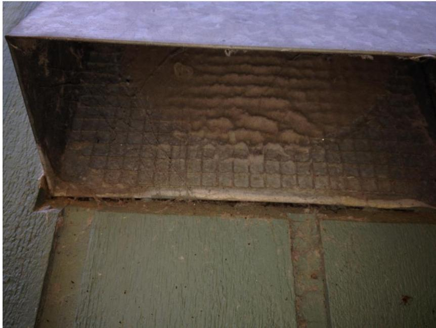
Figure 6: Obstructed combustion air supply ductwork (mechanical room ceiling)
