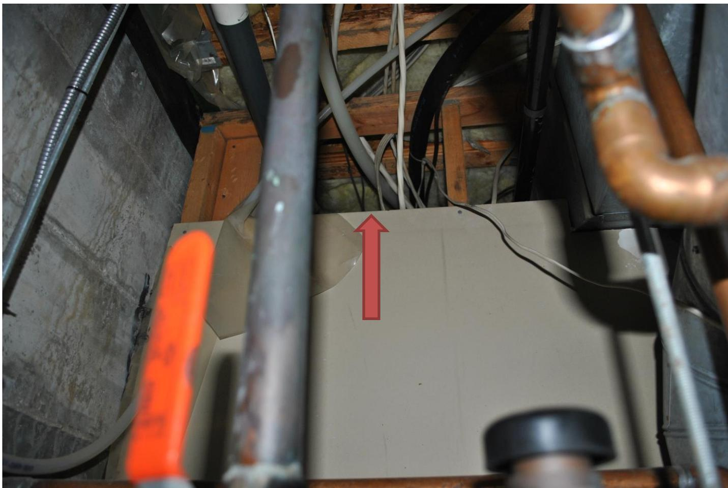
Figure 9: Return air ductwork in ceiling space and large unrestricted opening into ductwork
