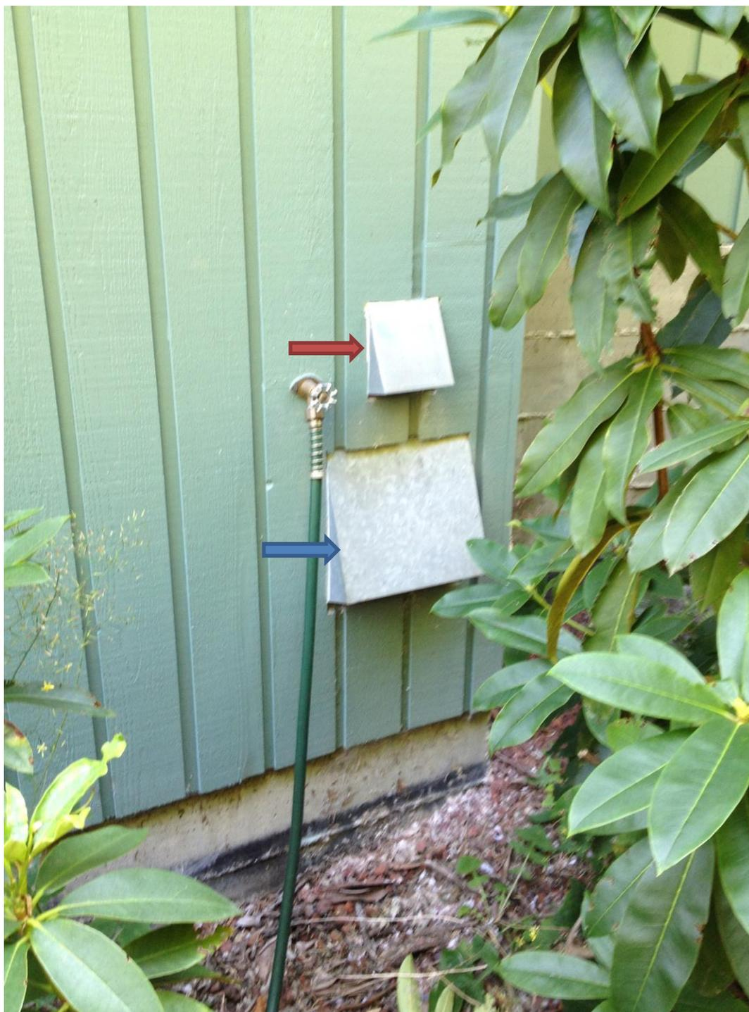
Figure 5: Blocked combustion air supply (outdoor termination)
