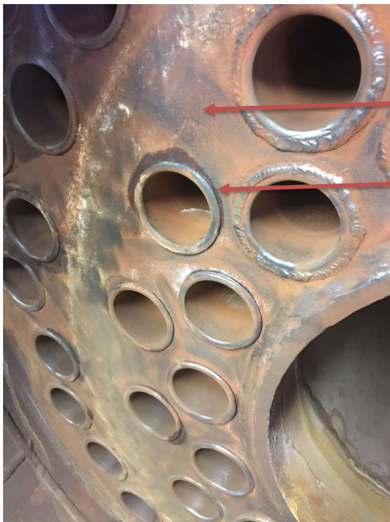
Closer view of leaking boiler tubes
