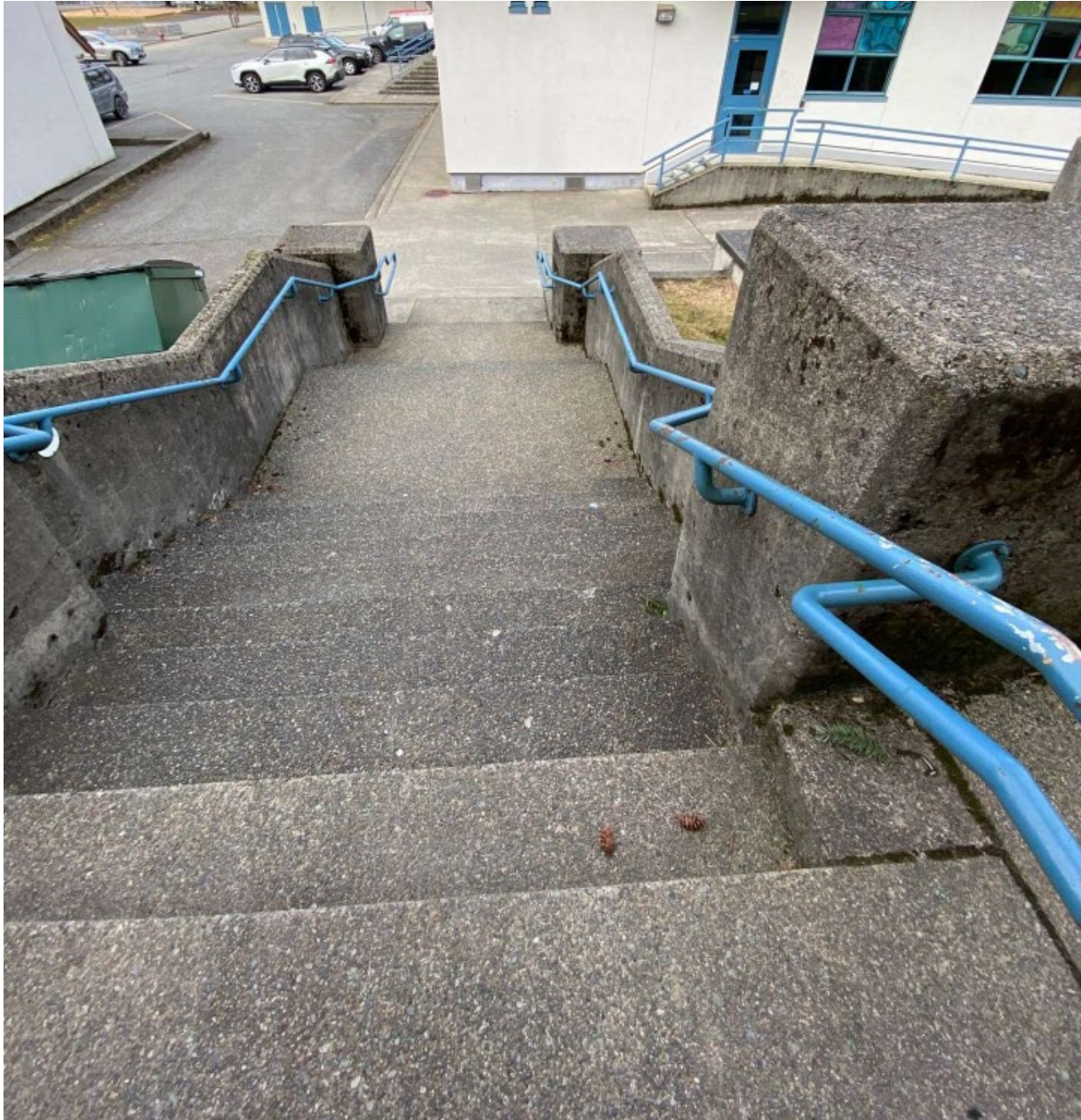
Image 1 - Stairs where the incident occurred.
