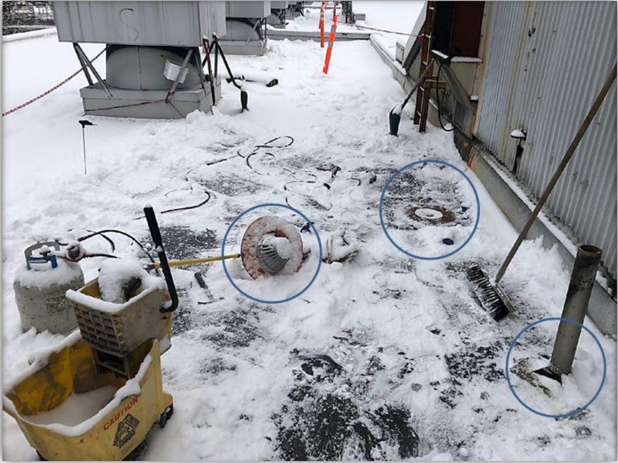
Photo 1 – Roofing components including roof drains and pipes.
