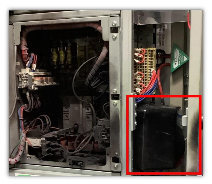
Image 6 – Inside the MCC bucket showing black soot resulting from the arc flash. [**BOX**] The point-to-point testing should have taken place on the de-energized load side conductors inside the raceway to the right of the MCC bucket.
