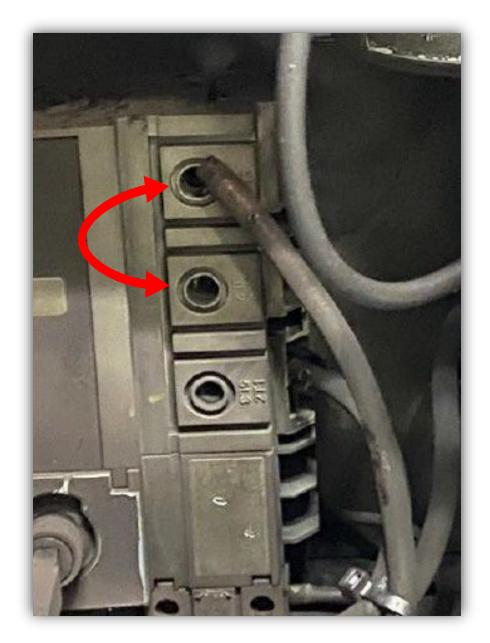
Image 8 – Closeup of line side breaker switch terminals. [Arrow] The energized line side terminals the electrician shorted out with the jumper wire causing an arc flash. Conductor melted and disconnected from terminal due to arc flash.
