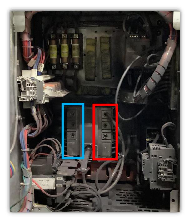
Image 7 – Inside the MCC bucket. [**LEFT**] The load side of the horizontally installed breaker switch (Deenergized when breaker switch open "off"). [**RIGHT**] The line side of the horizontally installed breaker switch (Energized when breaker switch open "off").
