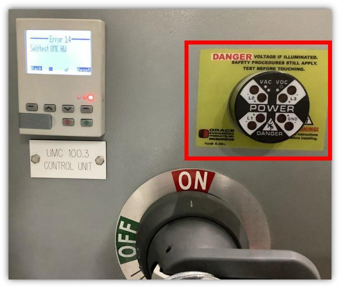
Image 4 – Closeup of MCC bucket door. [**BOX**] The through door voltage indicator identifying voltage on the load side of the breaker switch inside the cabinet.
