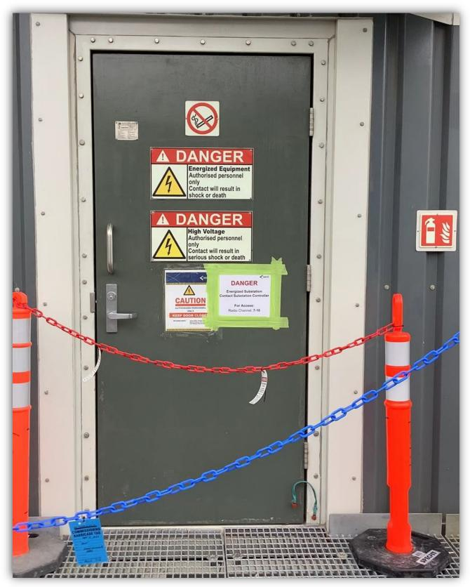
Image 1 – Access door into substation with warning signs.
