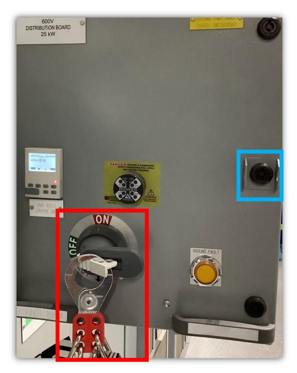
Image 3 – The MCC bucket door open. [**RED**] The lockout hasp with multiple locks affixed to the breaker switch, and rotary handle in the off position. [**BLUE**] One of three, quarter turned door latches that has a bracket allowing for a lock to prohibit opening of the door.
