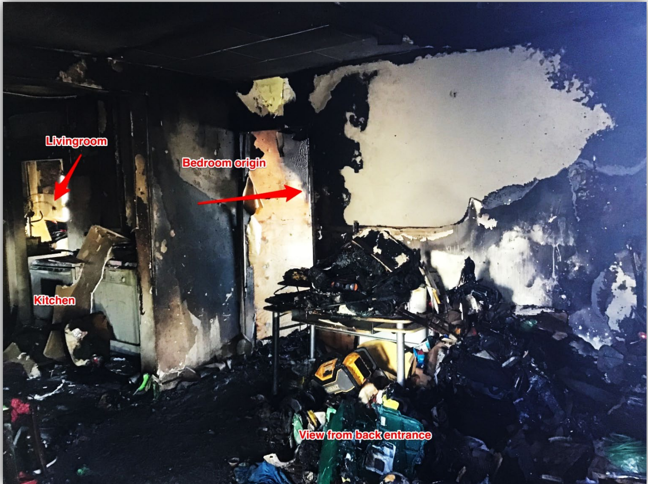
Photo 4 - Interior Southwards into mud room towards kitchen and bedroom/bathroom areas.
