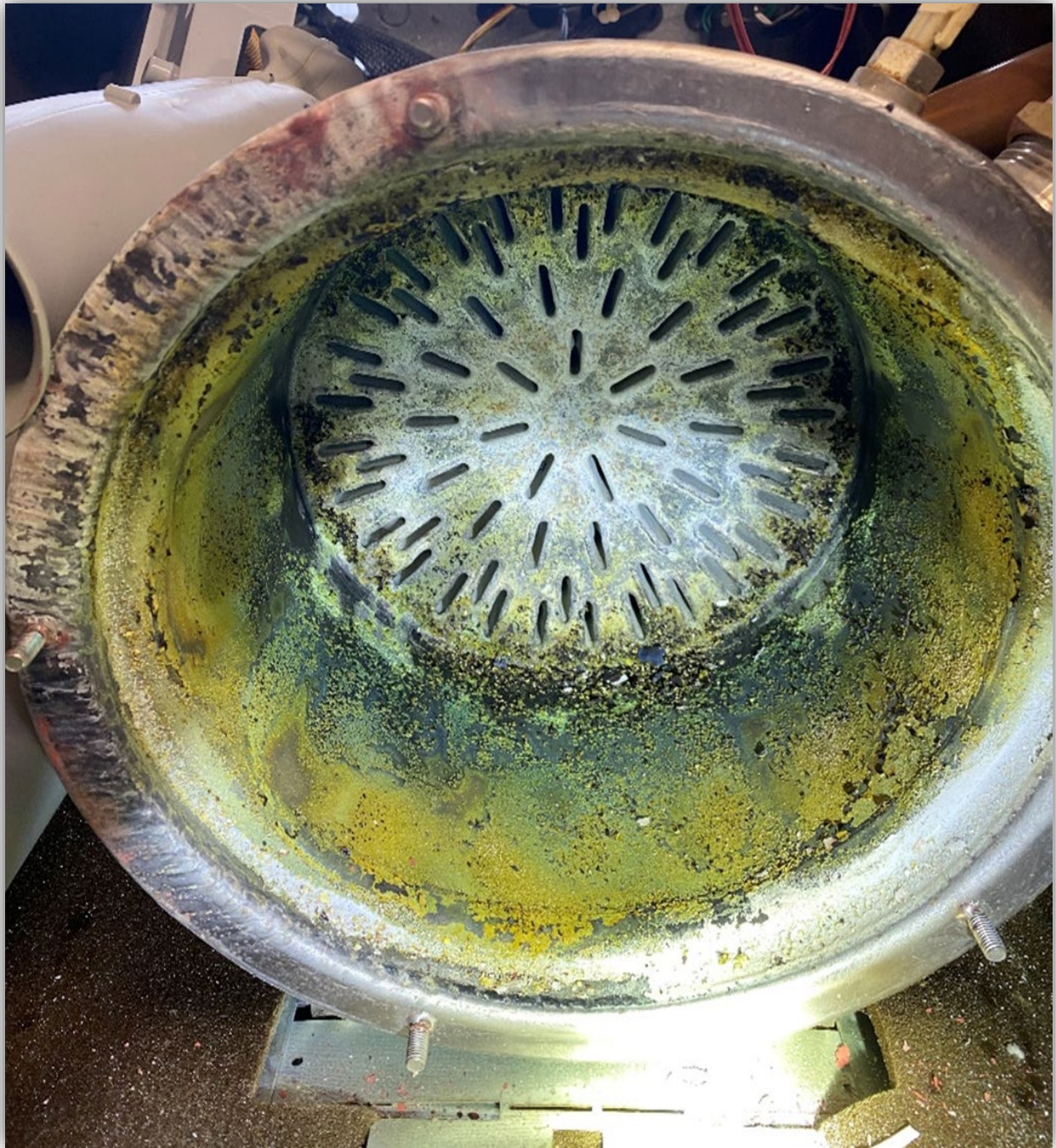
Image 2 - The inside of the heat exchanger.
