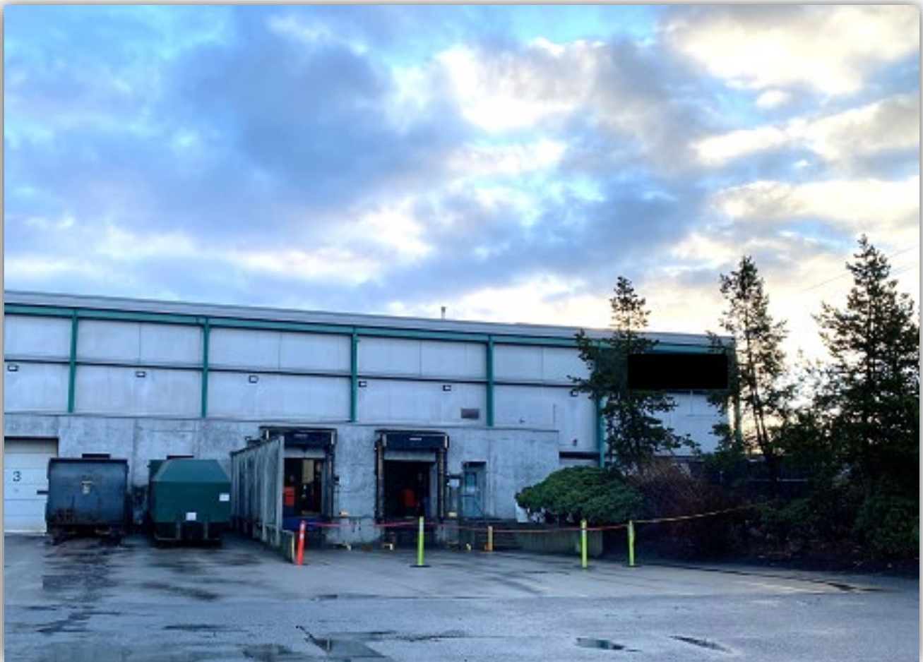
Photo 1 – Exterior of building's receiving area with two open bay doors for ammonia ventilation following the leak.
