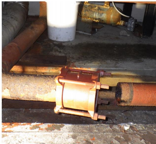
Figure 9: Separated brine coupling on 4" brine piping
