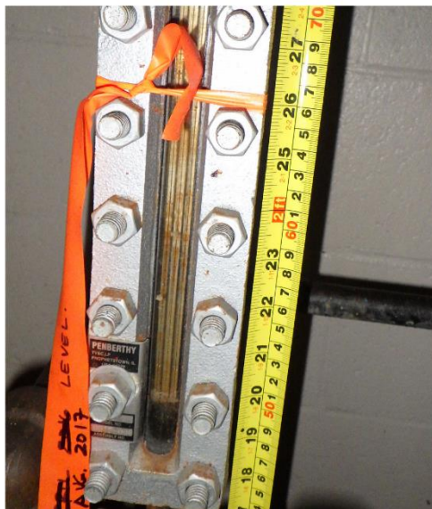
Figure 4: Indication of August 2017 receiver ammonia level.
