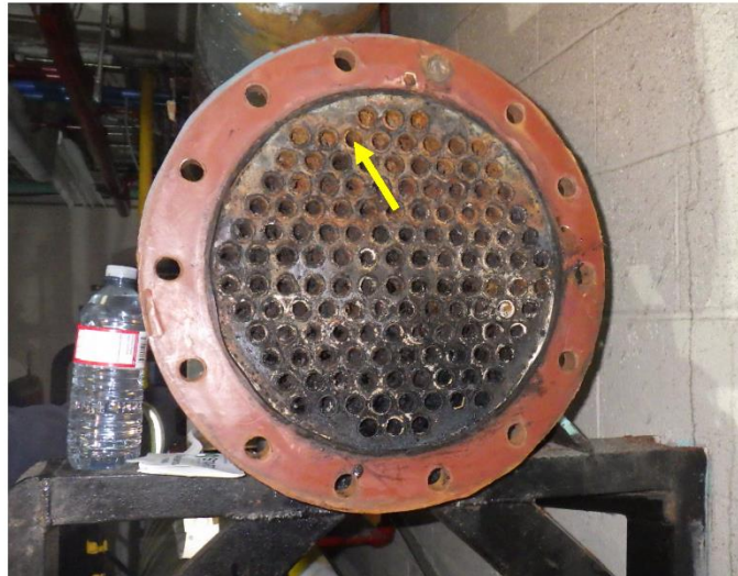
Figure 3: Return head of chiller showing clear tubes on upper half of the tube sheet and arrow indicating tube with leak
