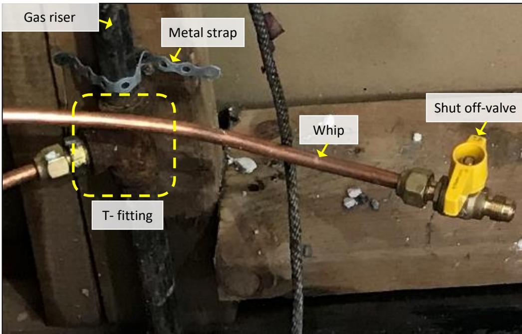
Photo 2: Gas riser pipe, T-fitting, copper whip and shut off valve in suite #2.
