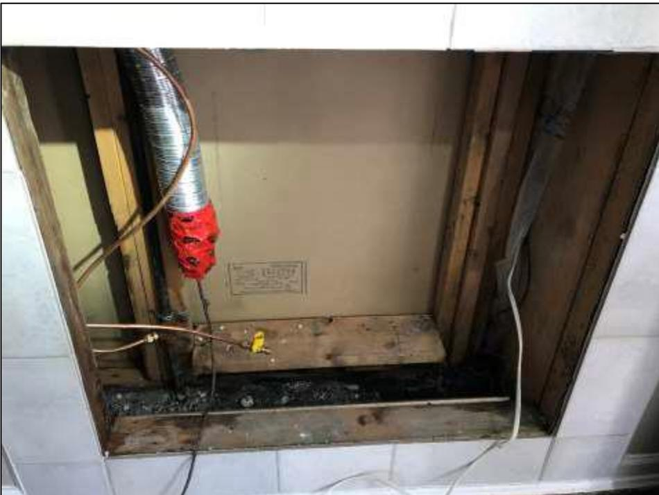
Photo 4: Gas fitting work completed to replace fireplace in suite #2 with a new whip and T-fitting moved left.
