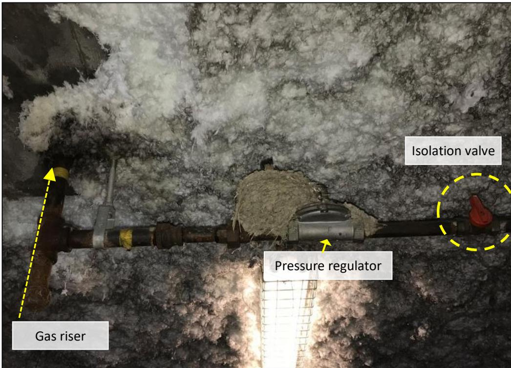
Photo 1: Gas line components located in the parkade: gas riser, pressure regulator and isolation valve which was turned “off” after the incident (as shown in photo).
