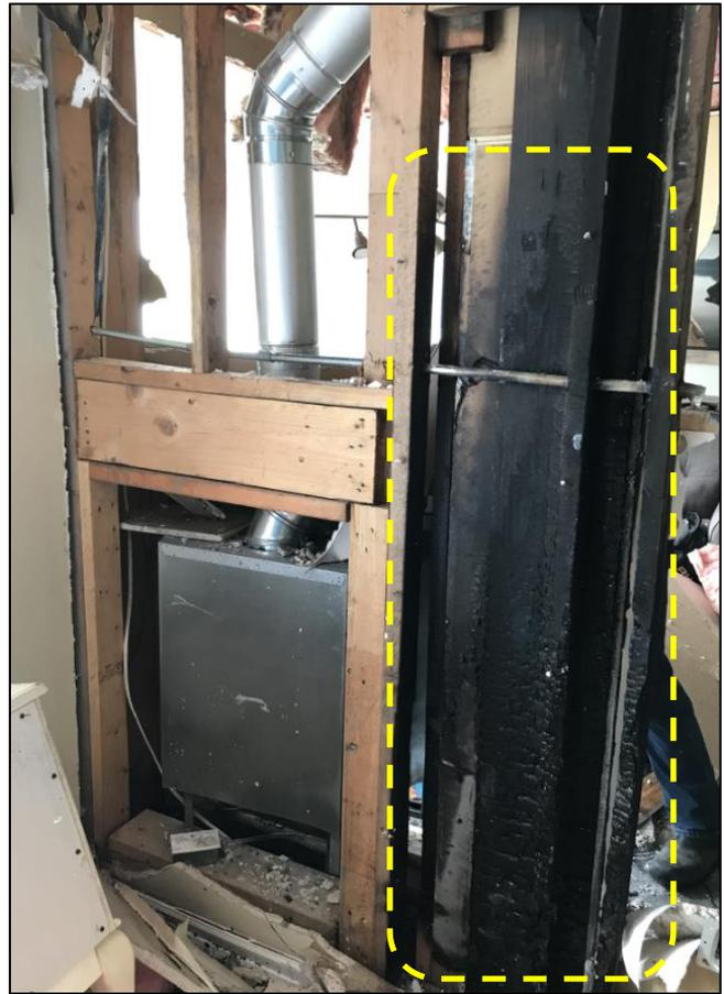
Photo 3 (a & b): (a) Fireplace in suite #3 partially blown out of wall. (b) Fire damage due to gas burning from broken whip.
