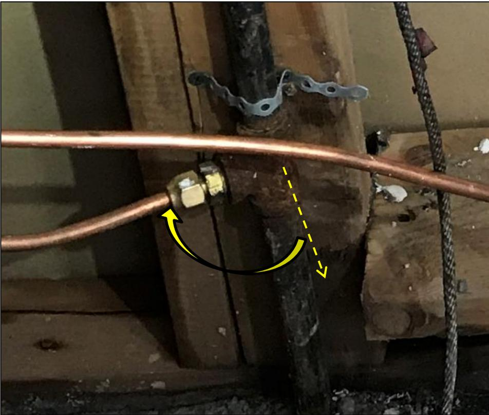
Photo 5: Gas riser T-fitting found moved and rotated in suite #2, as shown with new whip attached. The metal strap had been added by the gas fitter to restrain the riser pipe in its new position.
