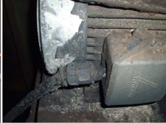
Photograph 7: P6 motor found with wire sheath not connected to the motor junction box.
