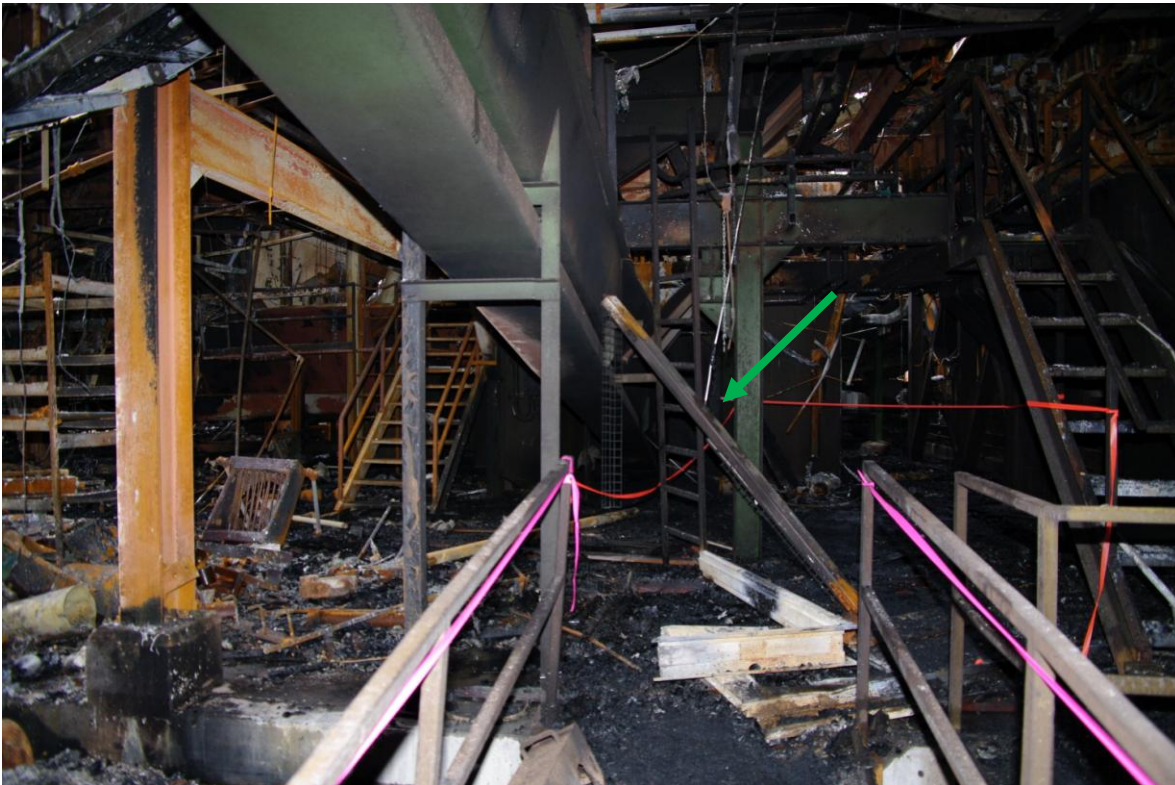
Photograph 44 Looking at examples of unprotected fluorescent lighting (arrow) (this and following photograph), grid J-23.
