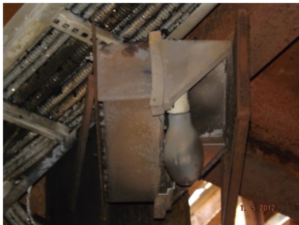
Photograph 12: Wall pack light assembly with missing cover found near the area of origin. The installed bulb is possibly a metal halide or high pressure sodium type.
