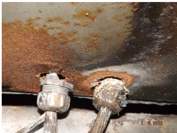
Photograph 19: Damaged neutral cables at the under-side of the transformer enclosure - external feed-through location.
