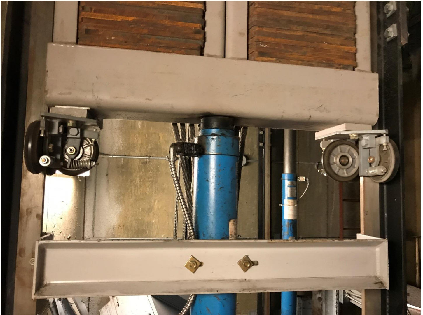
Figure 3- Counterweight buffer- fully compressed and bent due to impact of the counterweight. Counterweight frame bent.
