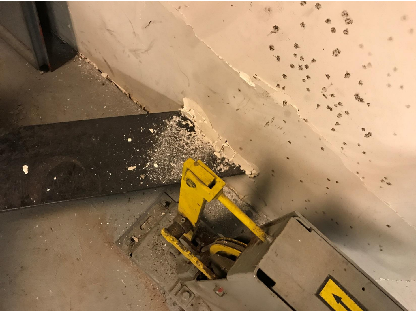
Figure 4- Machine beam in machine room. Machine beam dis-lodged due to impact.
