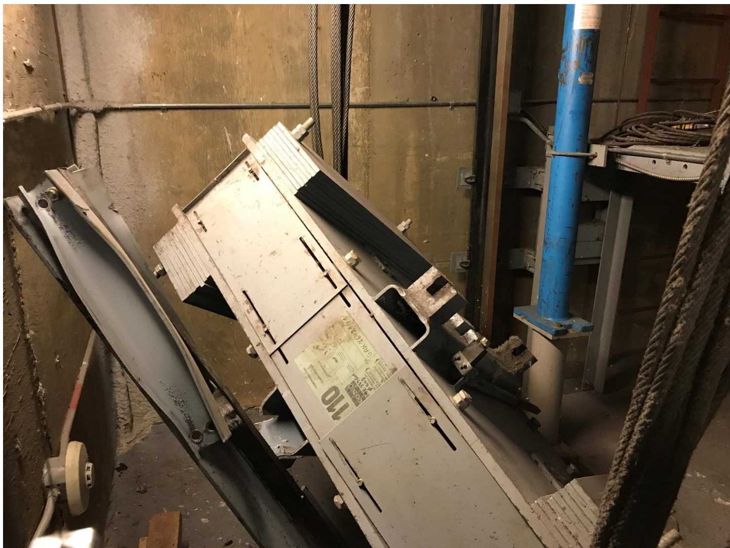
Figure #2- Mono –mass ( compensation rope tension device) mounting bracket torn from floor due to impact. Note slack ropes in the center rear of the photo tangled and damaged.
