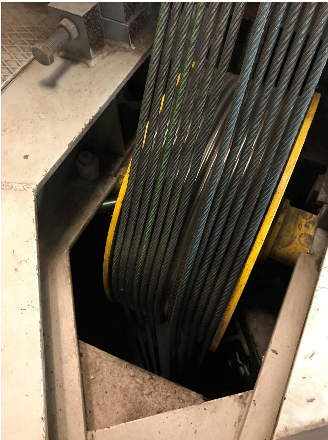
Figure 5- Secondary sheave with ropes displaced from sheave groove.
