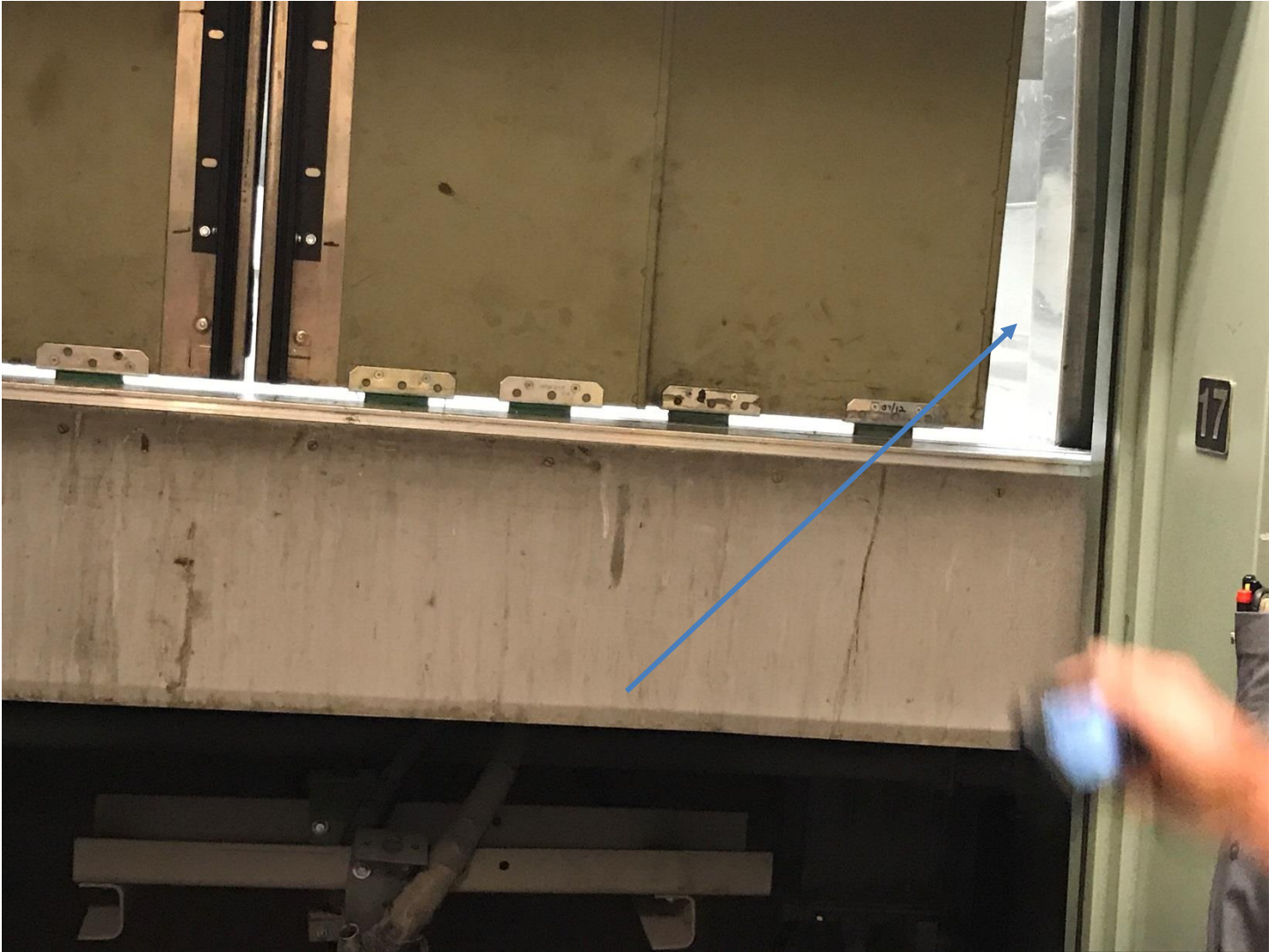
Figure 1- Elevator car above 17 floor landing. Arrow pointing at gap between car door and car door frame- Illustrates that amount of twist ( racking) sustained by elevator car due to impact.
