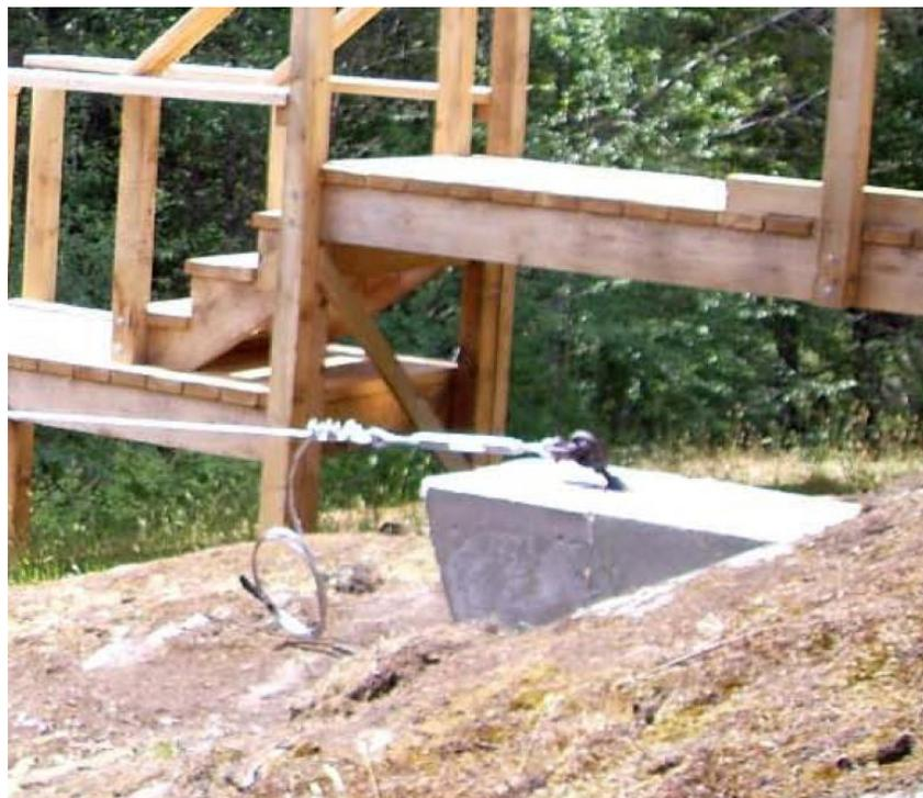
**Figure 2:** Side image of the zipline anchor and eyebolt in 2007 showing the angle between the applied load and the eyebolt threaded shaft
