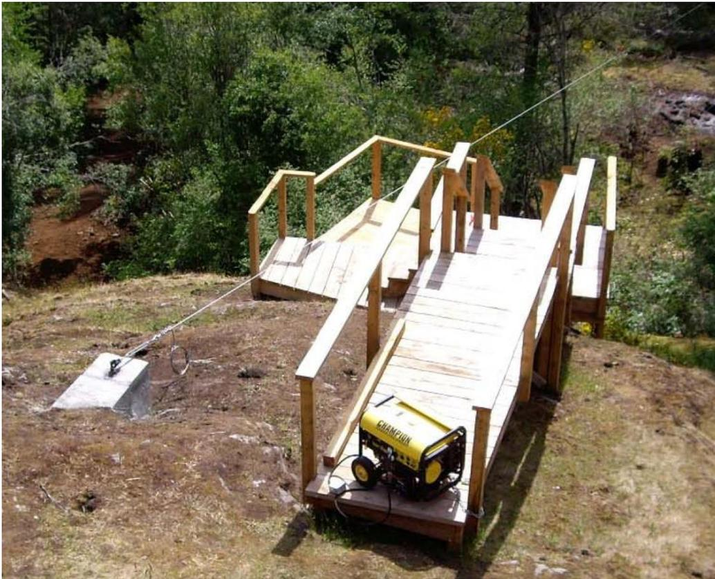
**Figure 1:** Overhead image of the installed zipline anchor and loading platform in 2007.
