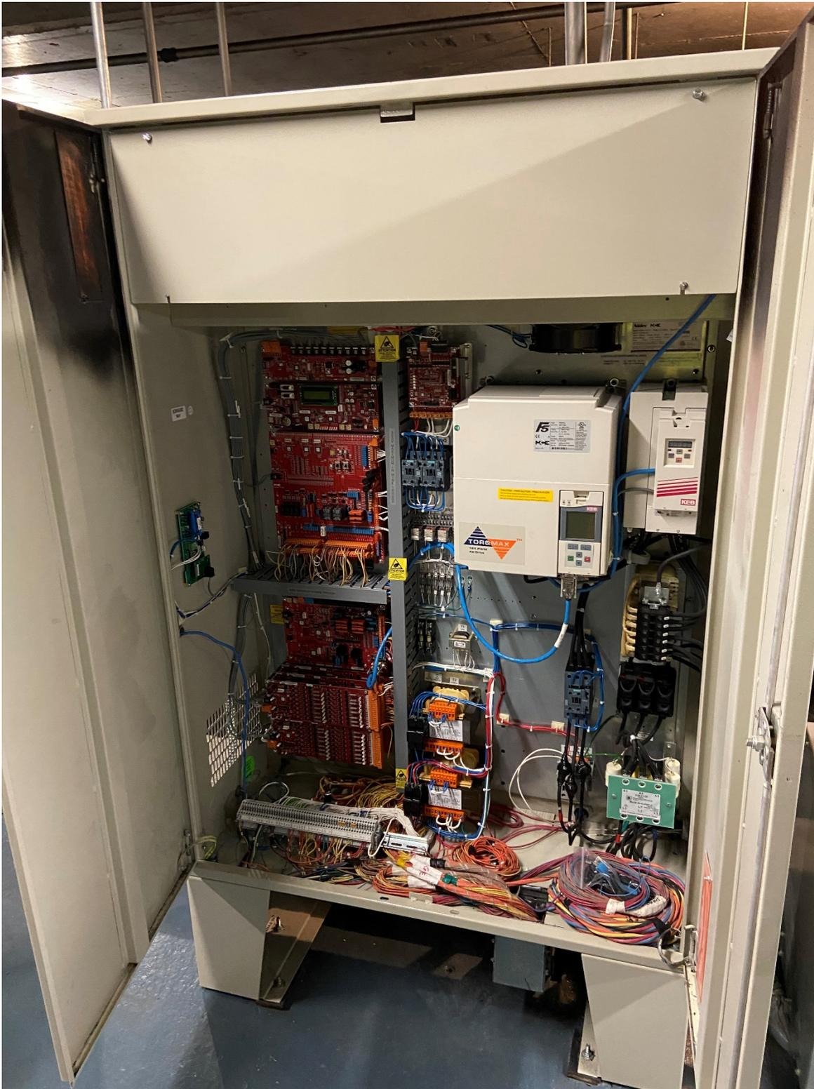
Figure 7 – Repaired Controller (Interior)
