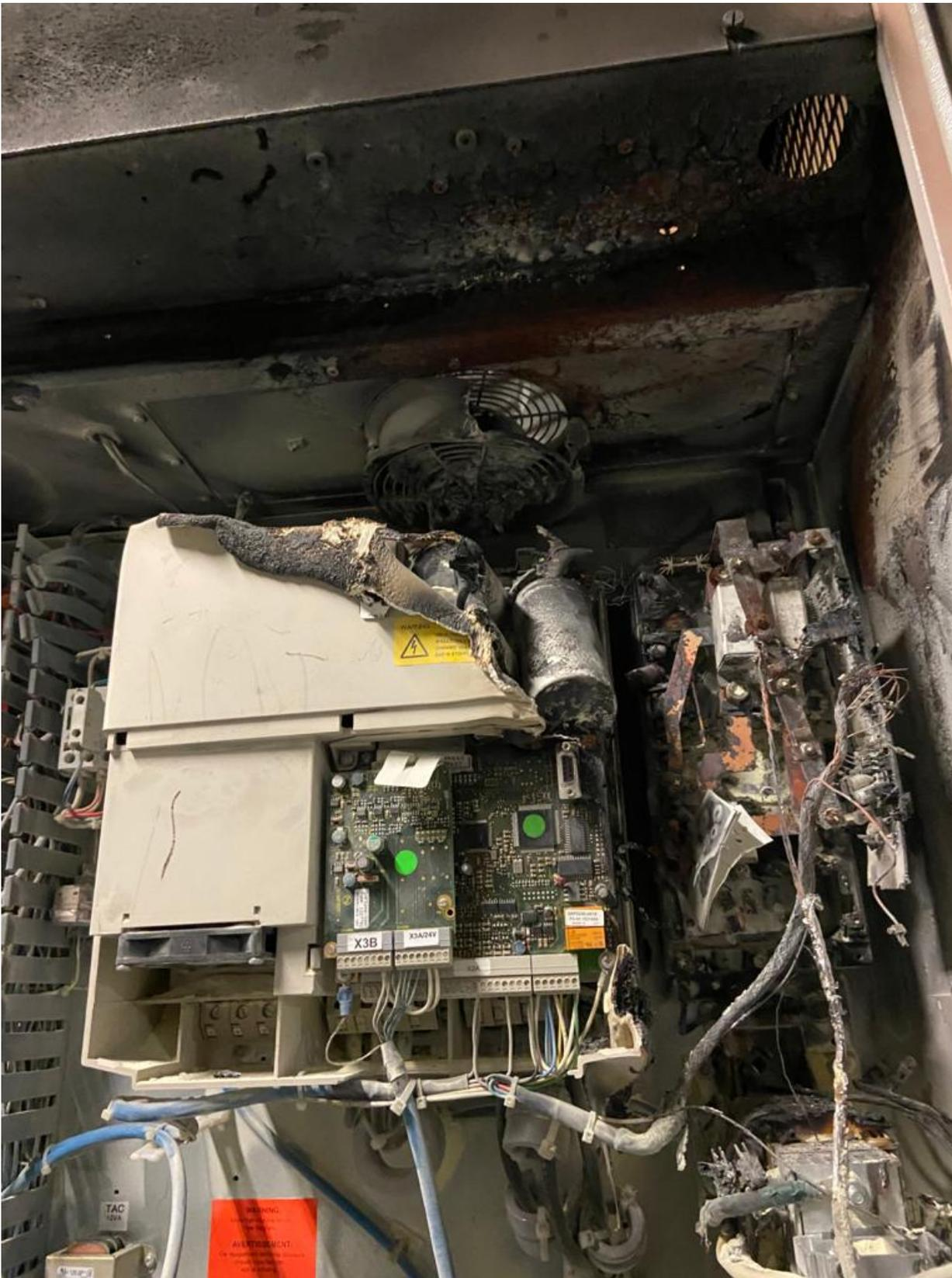
Figure 4 – Damage around VFD and Regenerative Drive Units
