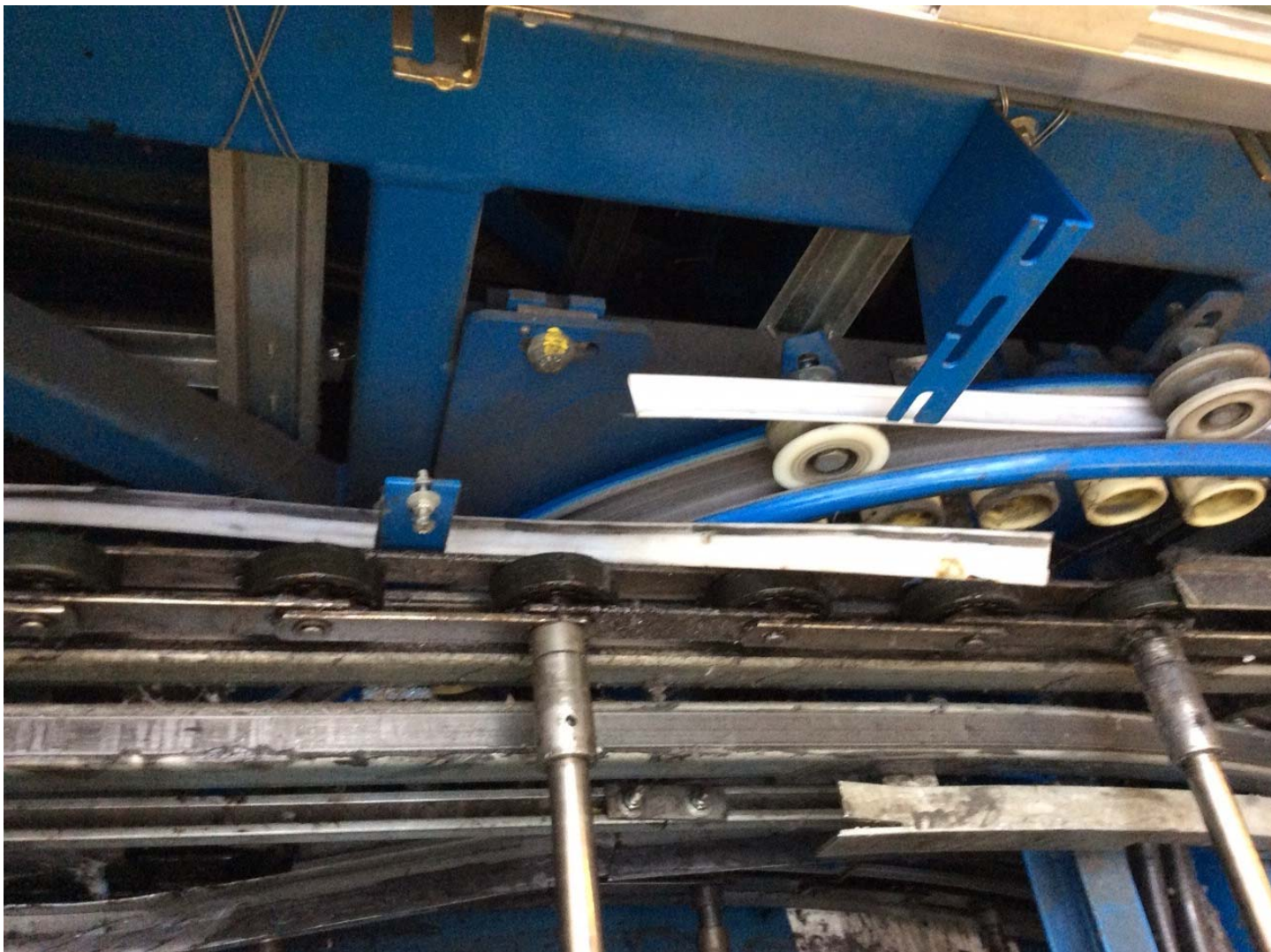
Handrail track pushed/pulled into handrail drive system.
