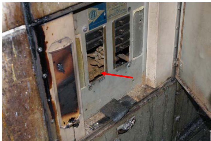
Photograph 3: Example of wood dust accumulation in MCC #9
