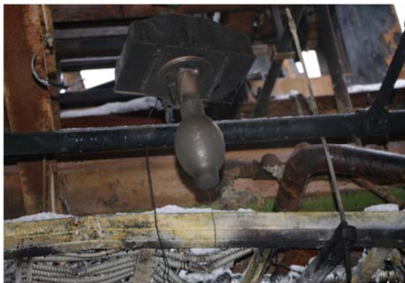
Photograph 6: Light assembly and metal halide bulb in front and above MCC #10
