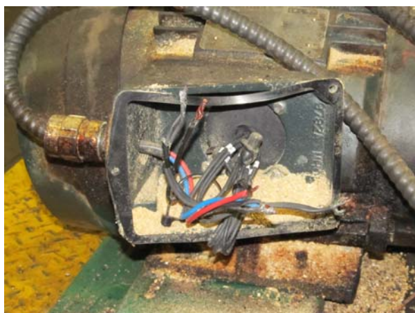
Photograph 8: Wood dust deposits within conveyor motor junction box labeled 8R-26.
