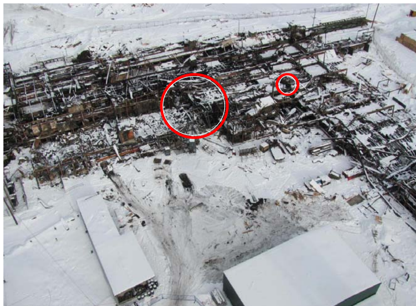
Photograph 2: Aerial view of the sawmill site after the explosion and fire of January 20, 2012. The circles indicate the possible areas within the basement where the explosion originated.
