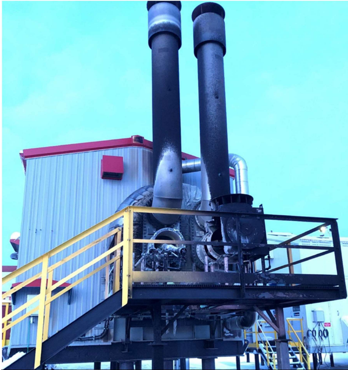
End View of Treater Firetube Burner Section
