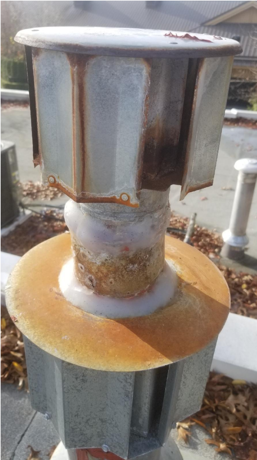
Figure 5. Picture of the vent cap.
