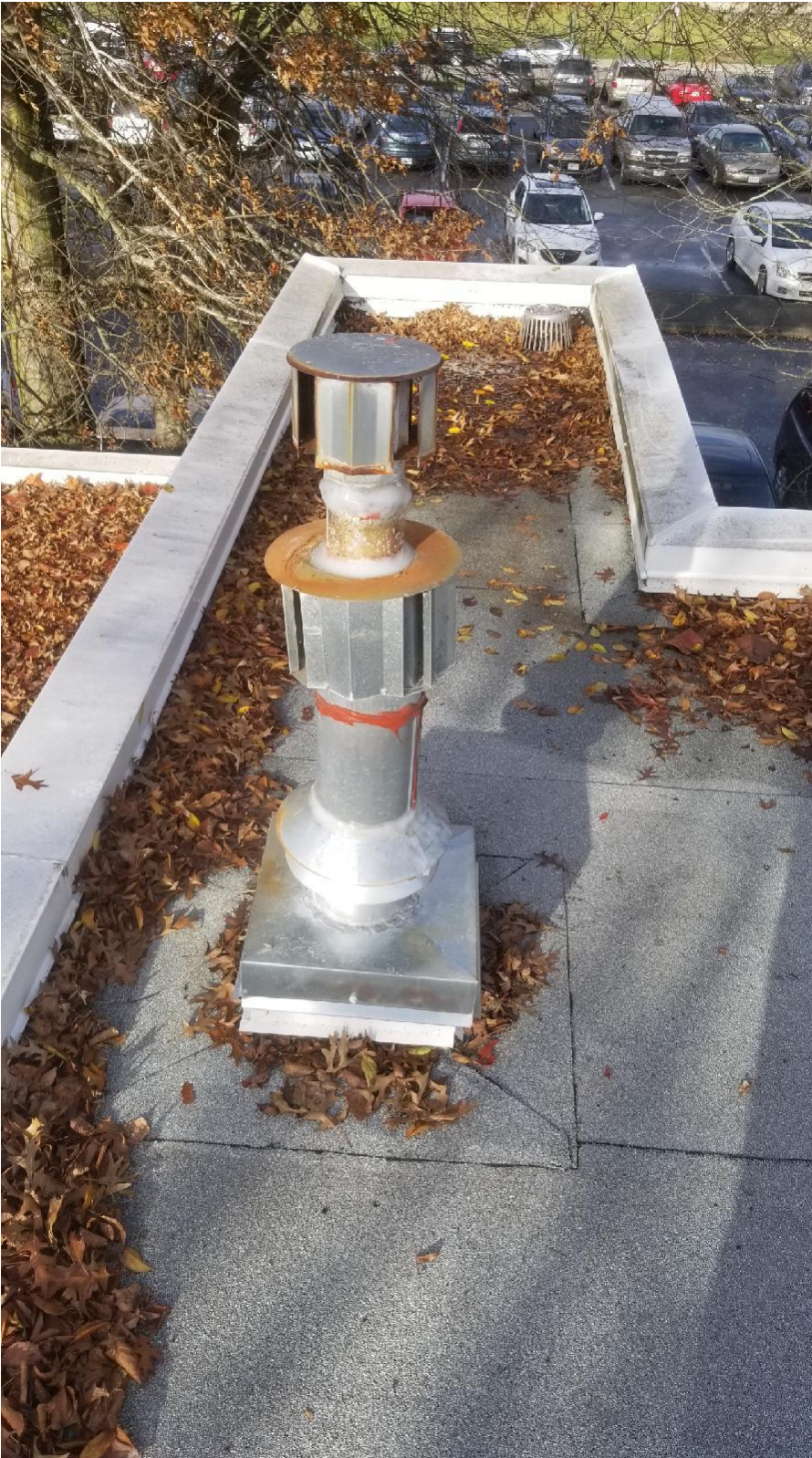
Figure 4. Appliance concentric termination. The top cap vents products of combustion. The bottom cap brings in fresh air for combustion.
