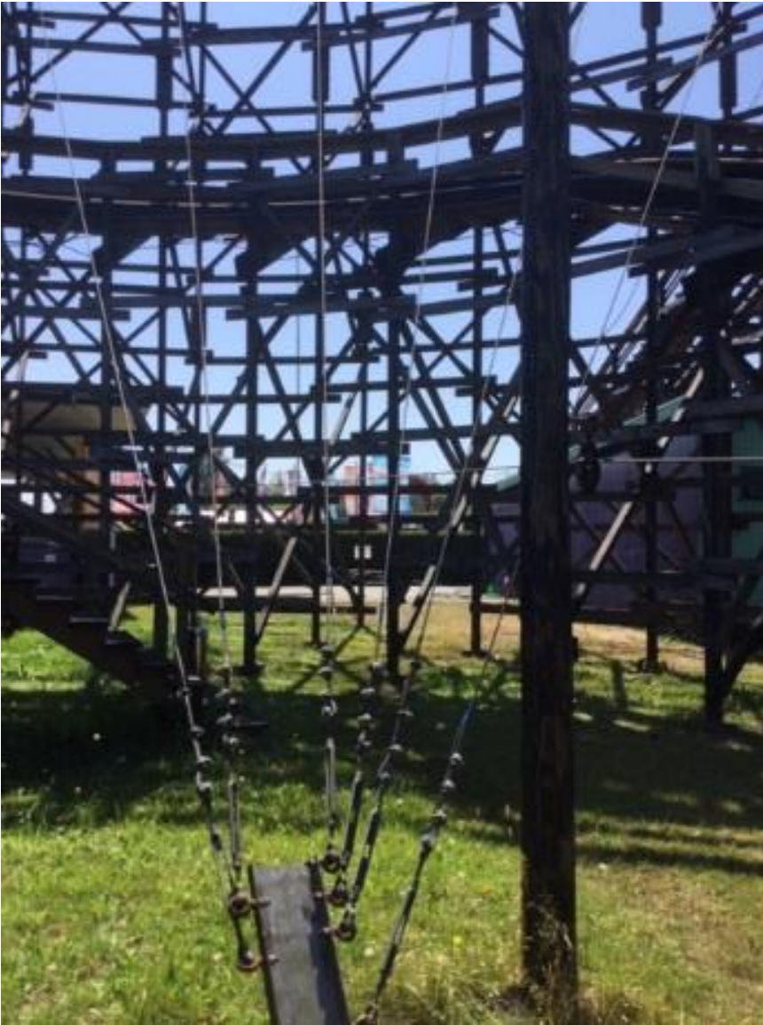
Photo 4: East guy lines connected to southern upper horseshoe.
