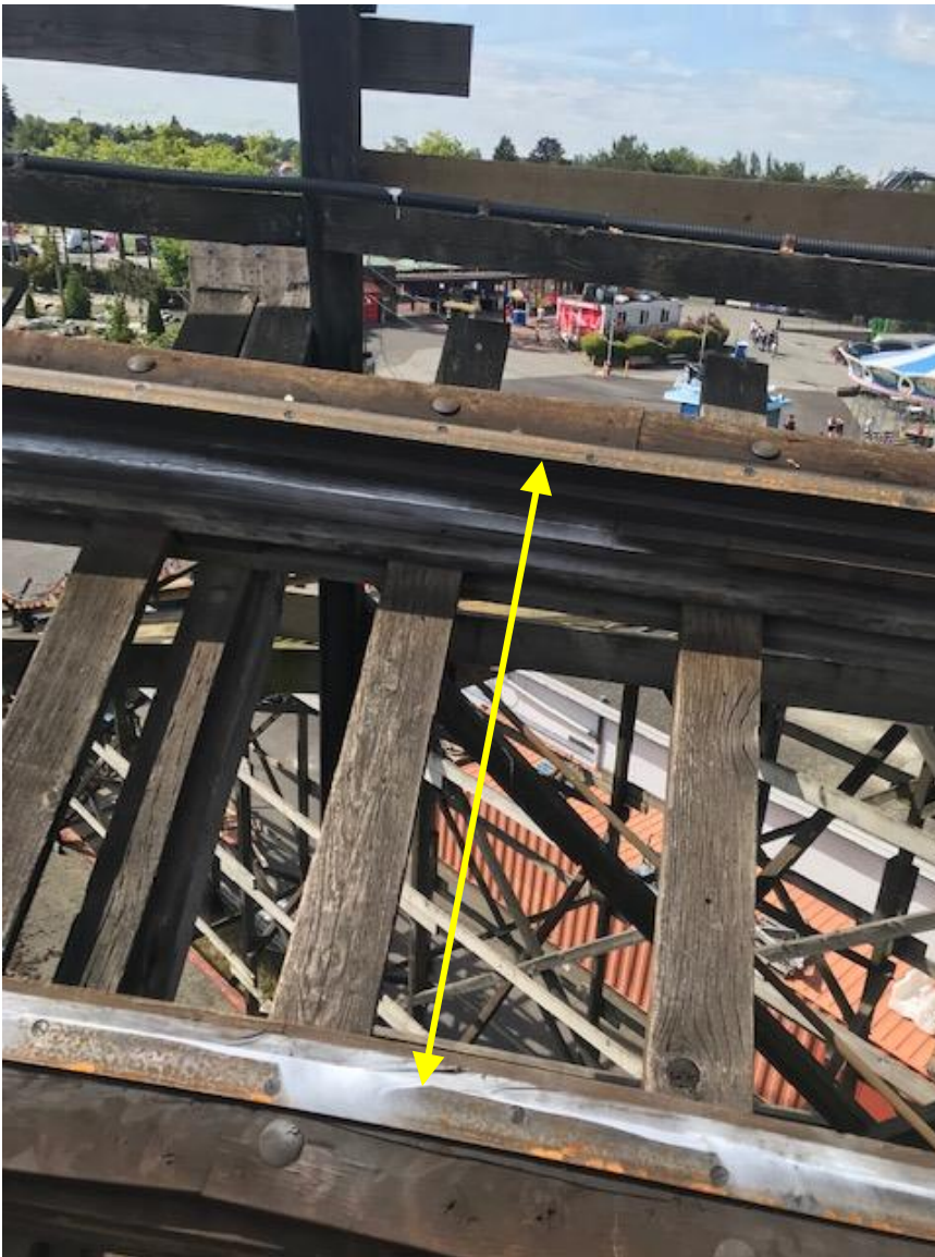
Photo 2: Track gauge width is the distance between the track steel rail plates, as shown above.
