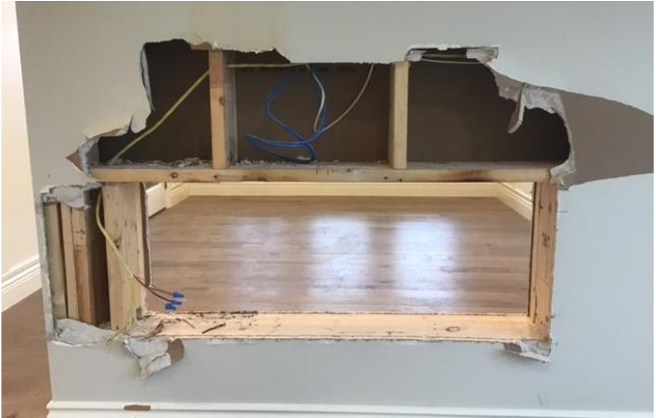
Photo 1: Location where the electric fireplace was installed.
