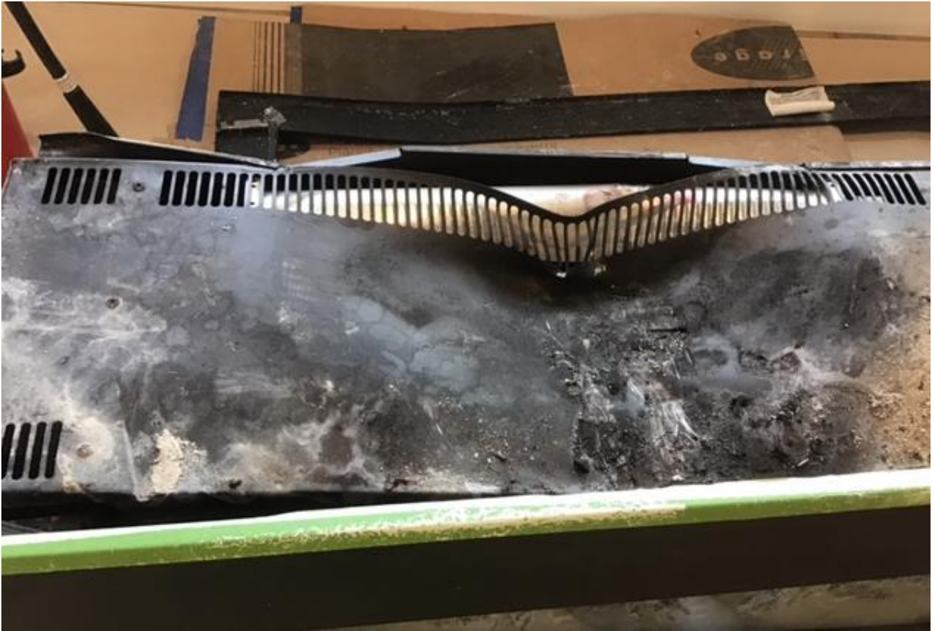
Photo 3: Damage to the top of fireplace.
